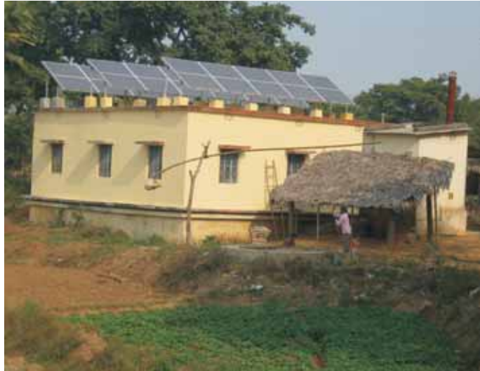
Power Station at Kurawa Village
