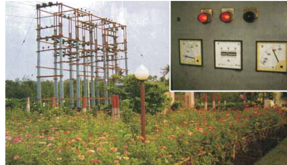
Transmission Lines to the Gasifier Plant
