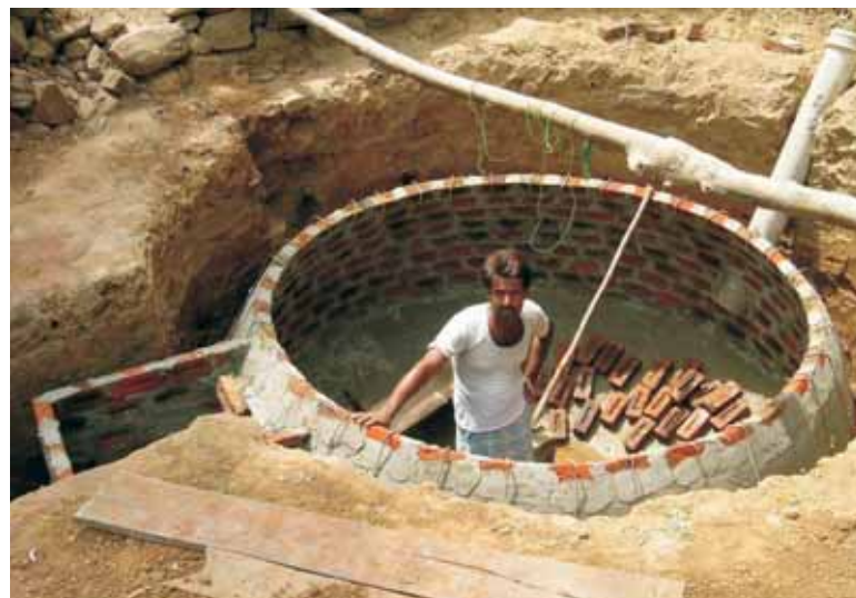
Construction Underway In Village Soorwal
