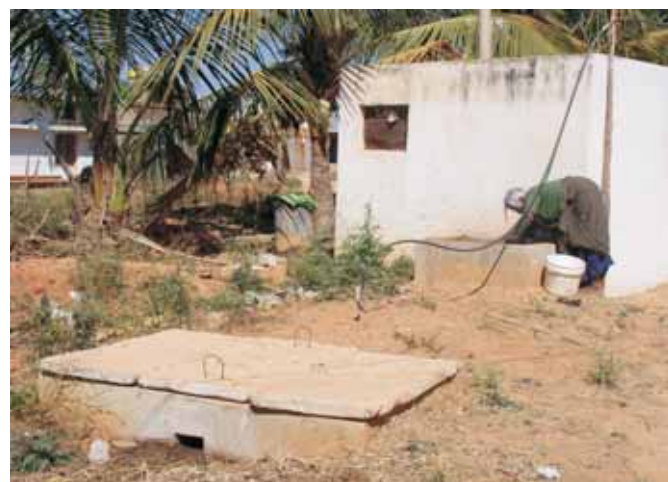
Feeding a Biogas Plant
