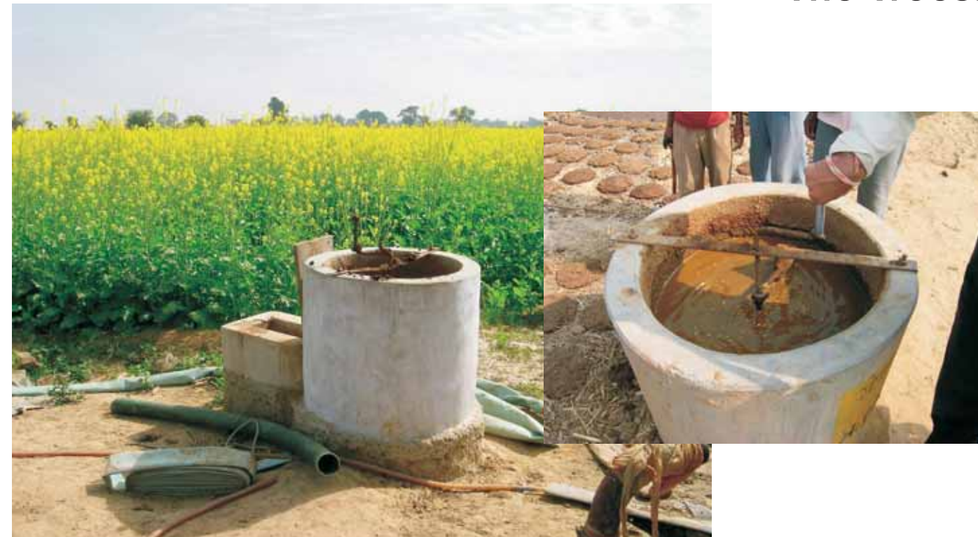
Biogas Mixing Tank
