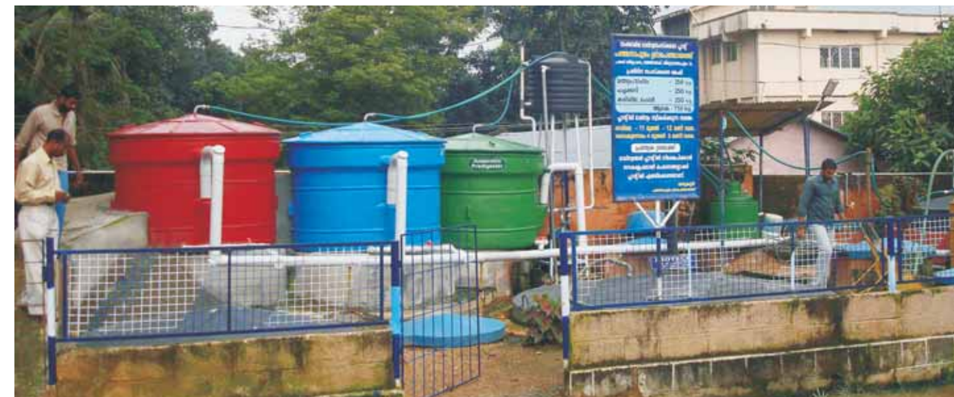
Biogas Unit in Patahanapuram
