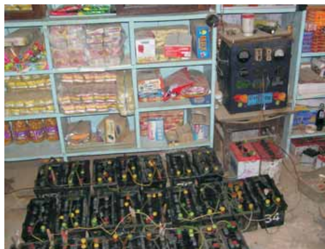
Battery Replaced with Electricity from SRE.
