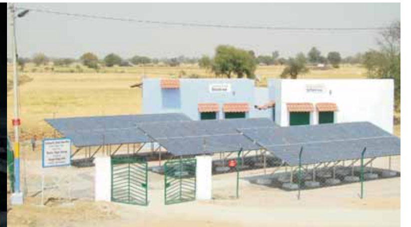
Community Power Plant at Rampura
