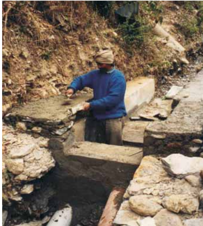
Construction of Flow Cannel for Water Mill Unit
