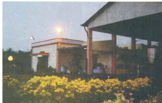
Illuminated in its Own Light: Gasifier Power Plant
