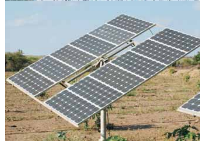
Solar PV Run Irrigation Pumps
