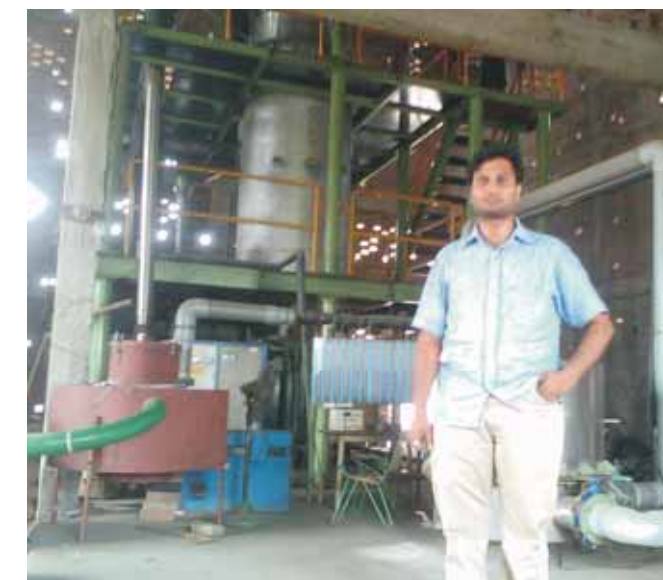
Biomass Power Plant
