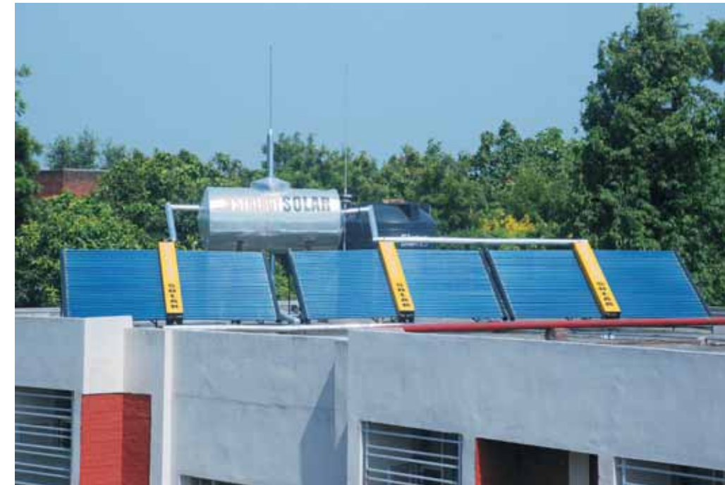
Solar Water Heater at MCM DAV College Hostel, Chandigarh
