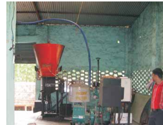
Biomass Gasifier at Gaiyari
