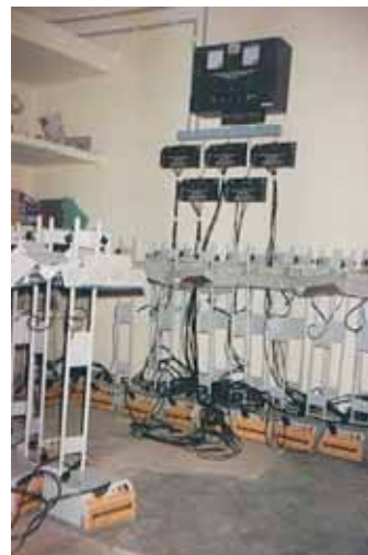
Solar Lantern Charging Unit
