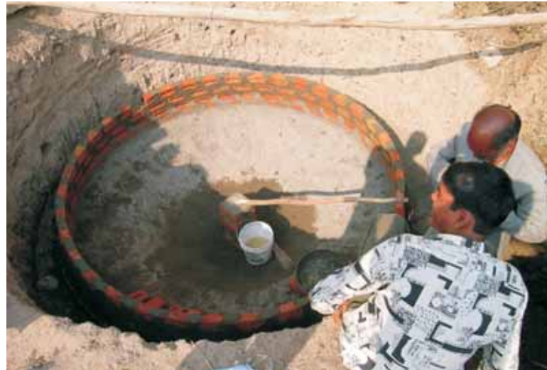
Digester Under Construction
