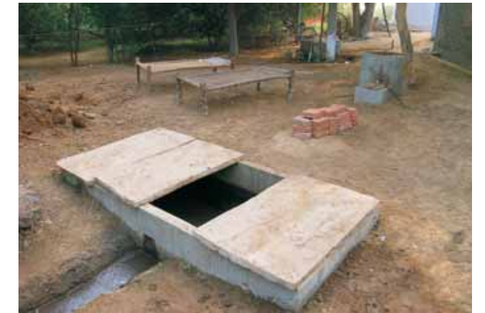
Covered Outlet Slurry Tank
