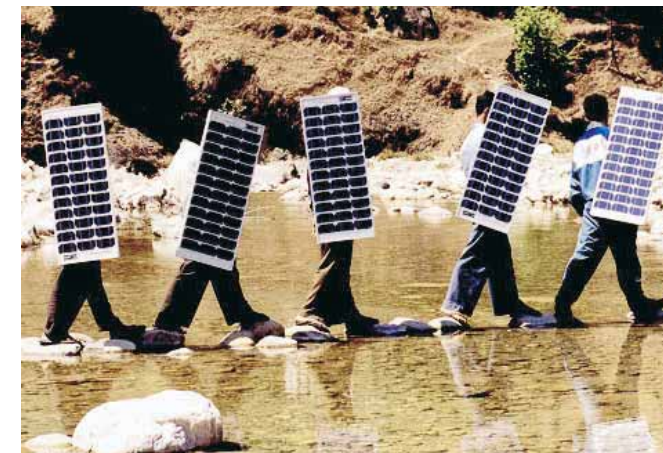
Installation of Solar Panels
