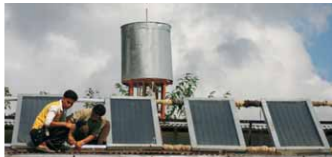
Solar Water Heater
