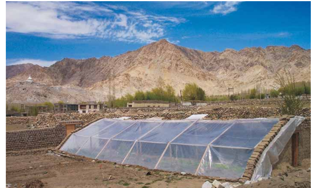
Solar Passive Greenhouse
