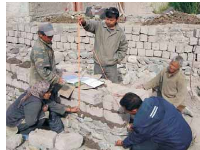
Construction of a Passive Solar Greenhouse at 14,000 feet
