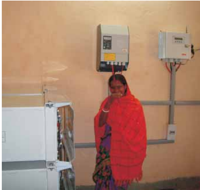
VEC Leader Inside Battery Room
