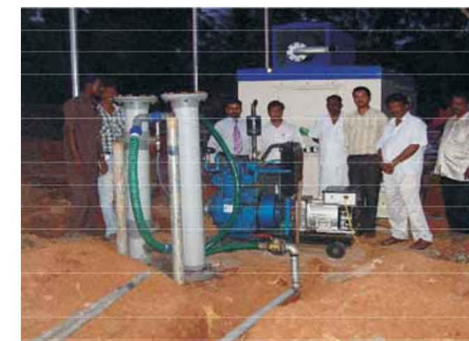
Proud Owners of Biogas Engine (10 kWh) with H 2 S Scrubber
