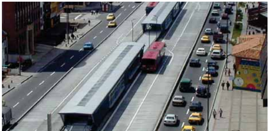
Bogota's TransMilenio BRT system with its bus stations and passing lanes.
