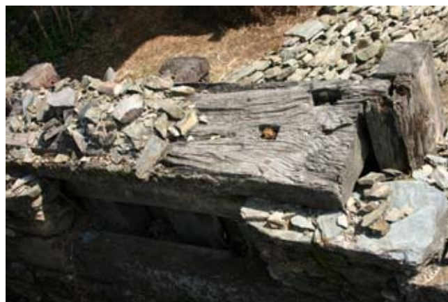
Figure 5. Housed and nailed joints used for fixing the wooden components of the Koti Banal architecture.
