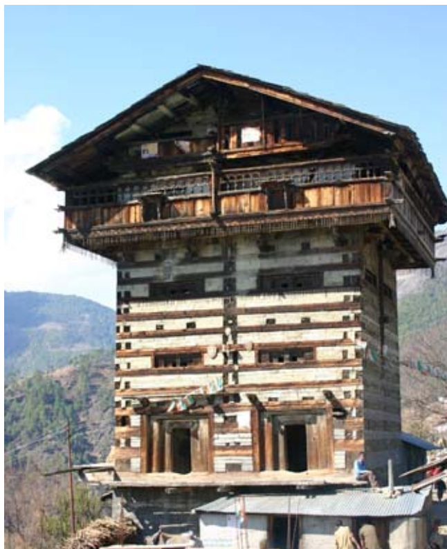
Figure 3. Five-storied structure of Koti Banal architecture constructed 880 \pm 90 yrs BP.
