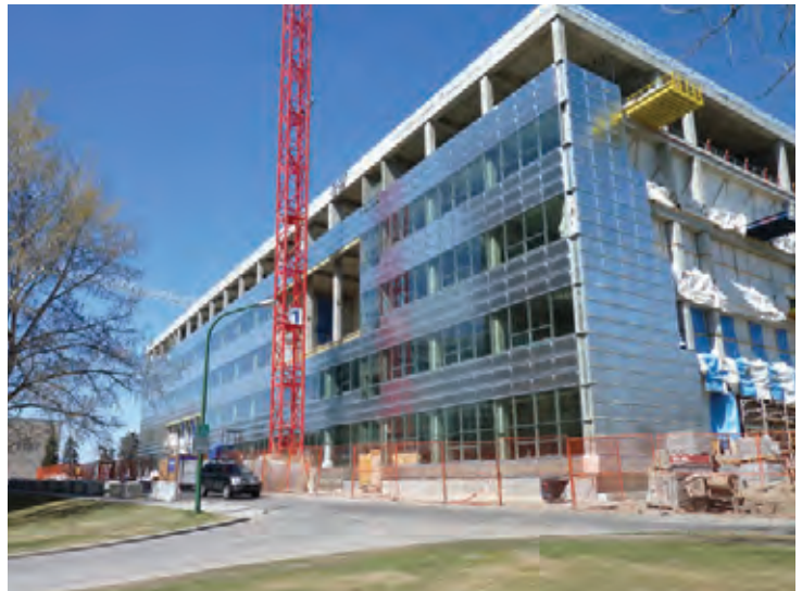
Energy Environment Experiential Learning (EEEL) Building, University of Calgary, Canada
