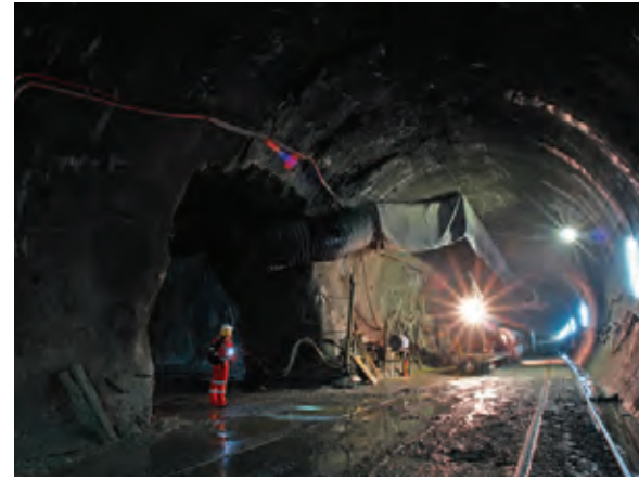
Gotthard Tunnel Construction Works, Switzerland
