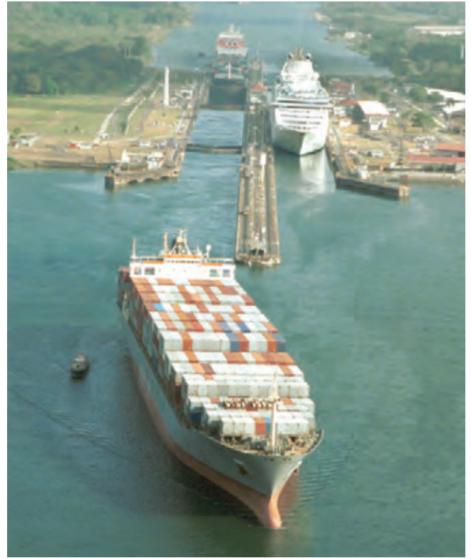
Panama Canal, Panama
