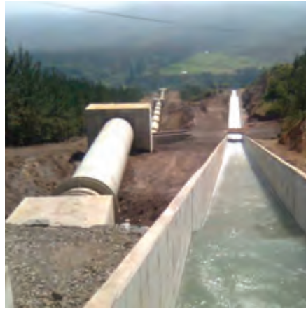
Hidromaule Lircay Project, Chile
