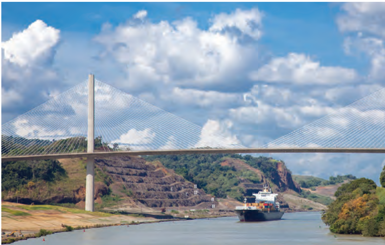
Panama Canal, Panama
