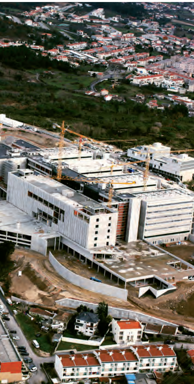
Braga Hospital, Portugal
