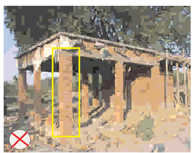
Never rest roof on unreinforced brick piers.
