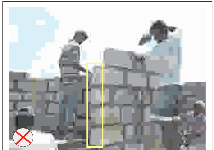
Never use thin concrete blocks in vertical position. They will make unstable wall.
