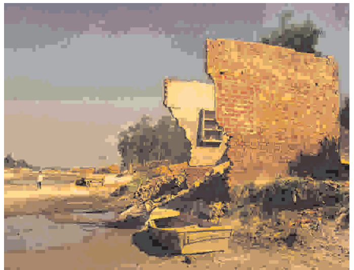
Wall collapse due to tidal surge
