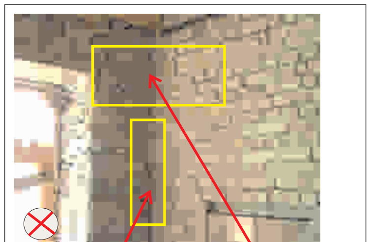
Never make inner wall without RC Band that is integrally connected to the Band in outer walls.
