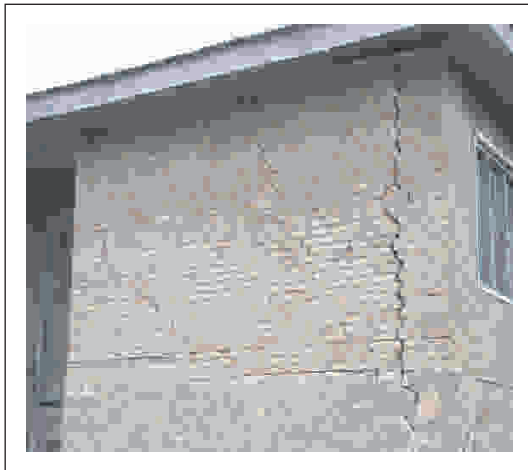
Large cracks
