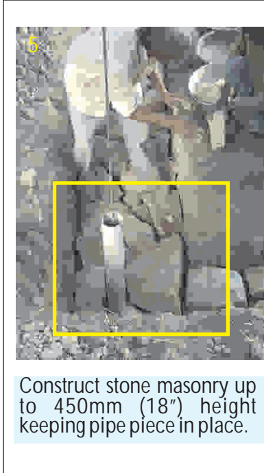
Pull out the pipe and fill up the cavity with 1:1½:3 micro concrete for Zone IV & V and 1:2:4 micro concrete for Zone III while continuously rodding. Ensure min.50mm (2") concrete all around the bar. Put back pipe in place and continue with masonry construction around it.
