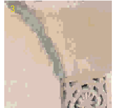
3 Fill up the gap with 1:3 Cement mortar. Finish the restored parts to match the surrounding wall.
