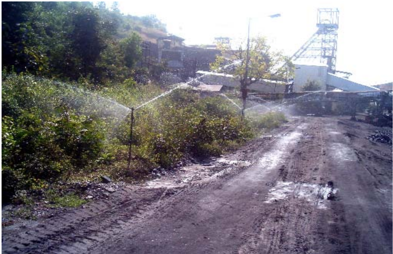
Figure 4.1.6 - I: Water Sprinkling for Dust Minimization
