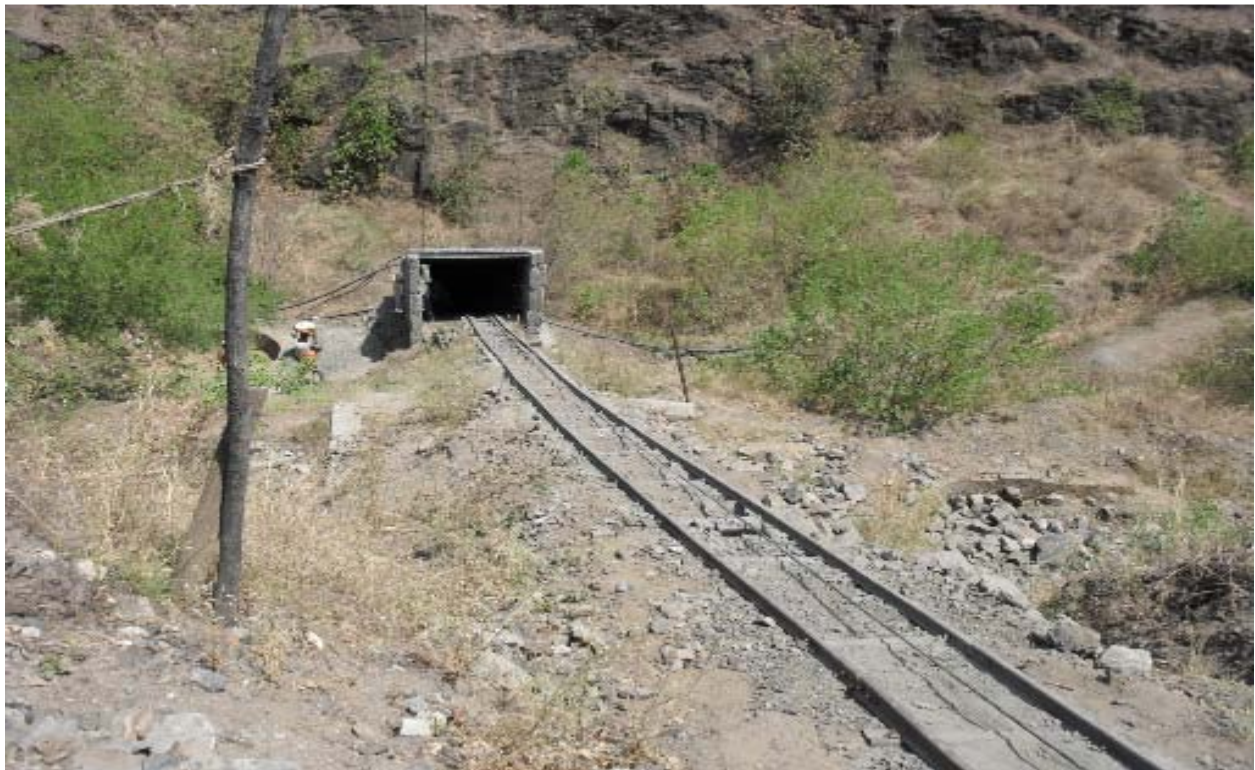
Figure 4.1.5 - I: Sonewadi Underground Mine
