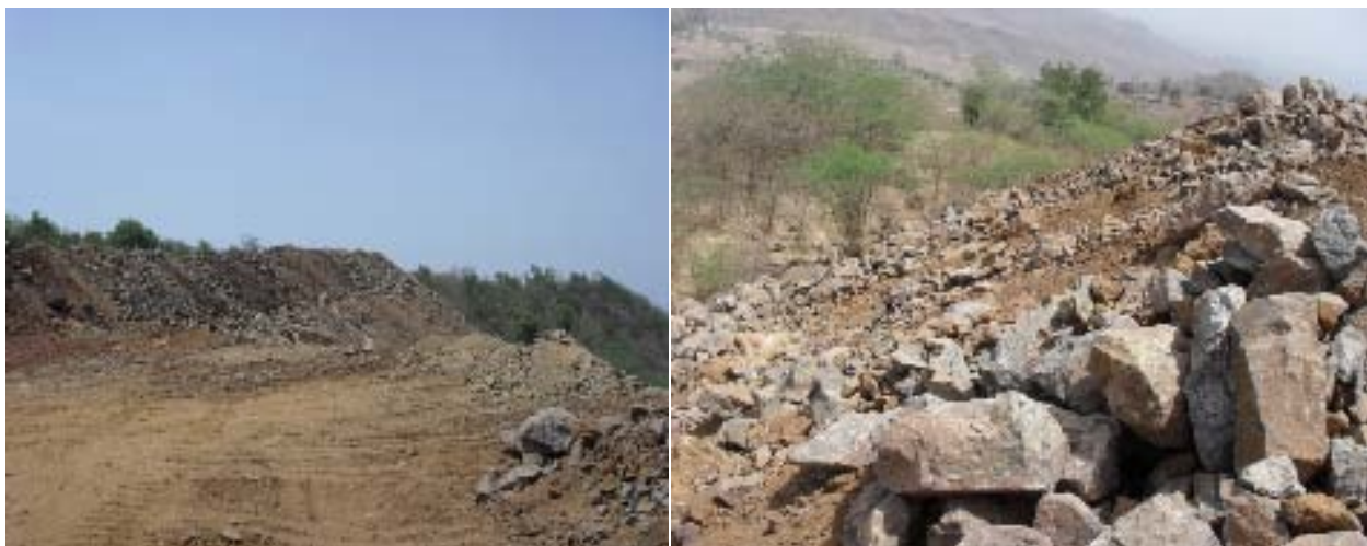
Figure 4.1.11 - III: Dumps not stabilized
