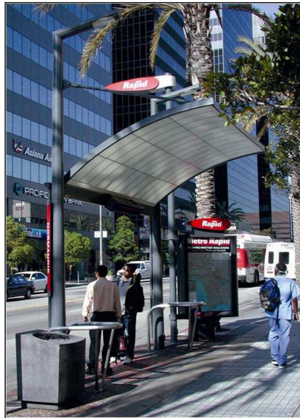
FIGURE 2.5 – Metro Rapid Canopy
