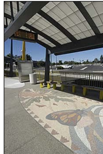
FIGURE 2.8 -Terrazzo Paving at Station
