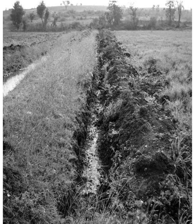
**Fig. 16: Drainage Channels for Seepage**
