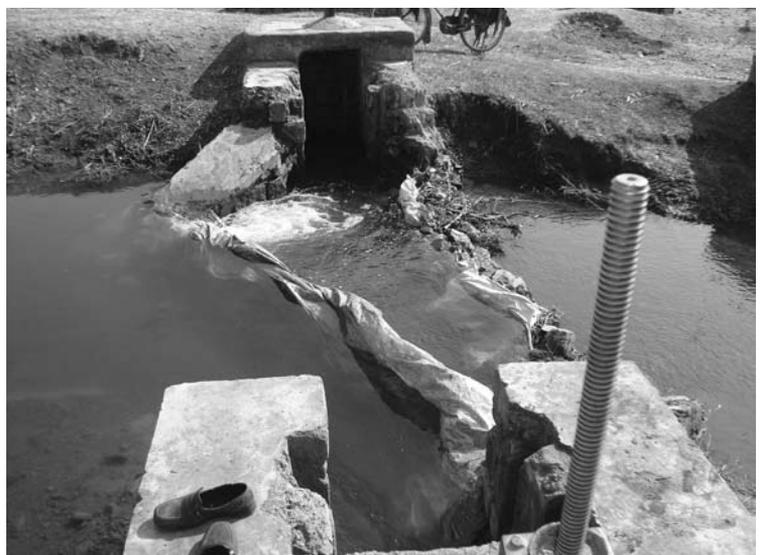
**Fig. 17: Impromptu Bunds on the Main Canal Diverting of Water into Distributaries**
