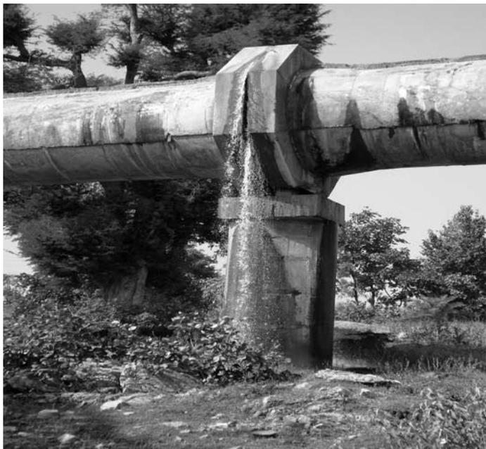
**Fig. 9: Leaking Aqueduct**
