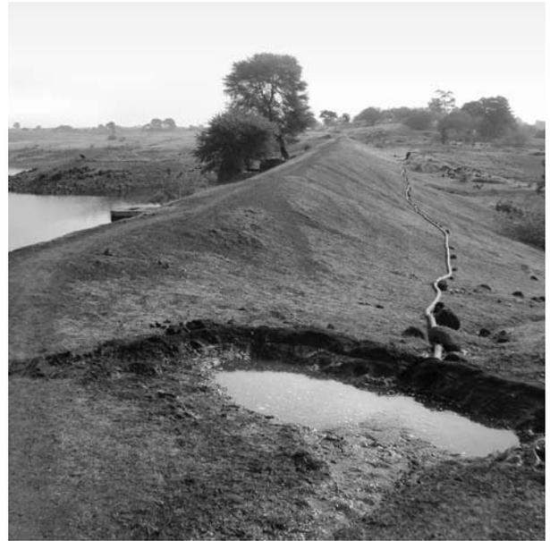
**Fig. 12: Diverting Seepage Water for Irrigation**
