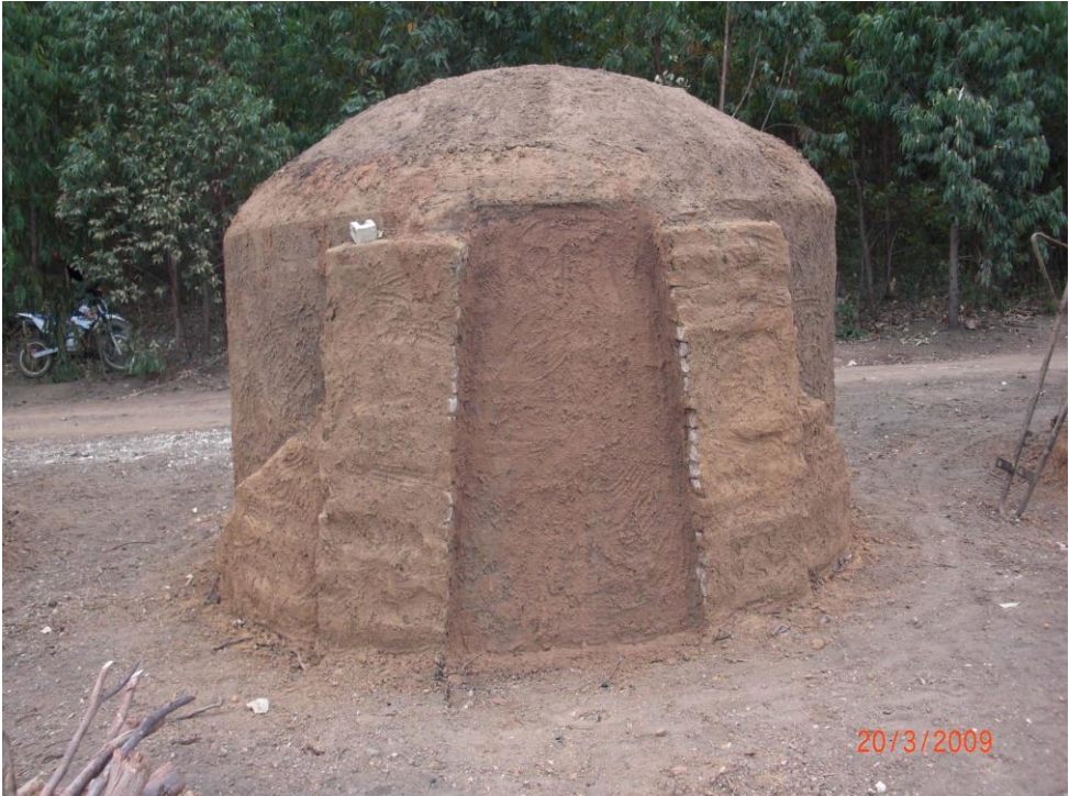
Photo 17: Low cost brick kiln for charcoal production in Minas Gerais.
