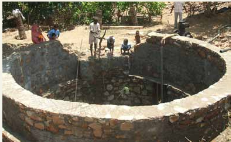
Well cleaning work under progress on another well in Dhala
