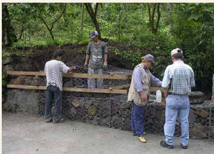
Roadside retention wall in Berlín
