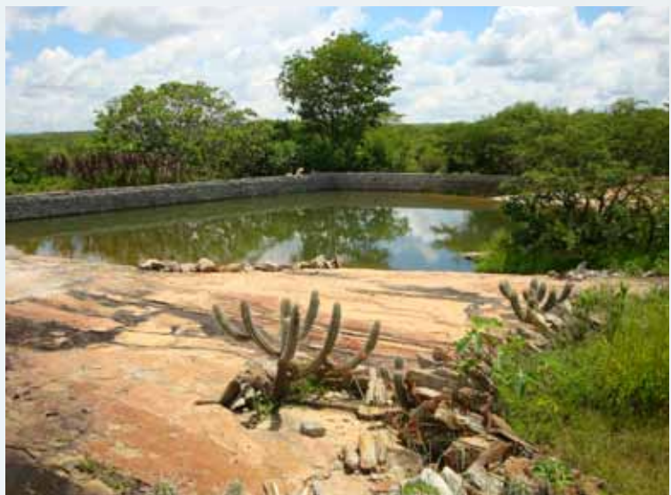
Dams are sited where there are natural embedded rocks, which are then surrounded by a brick wall, making the water accumulate
