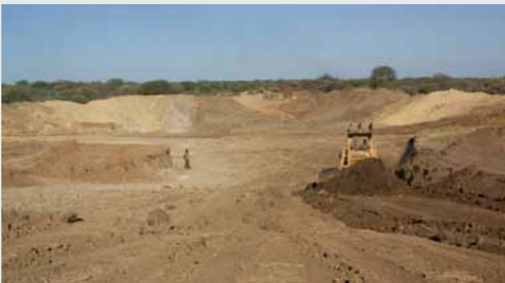
Pond construction in Dawe Kachen District
