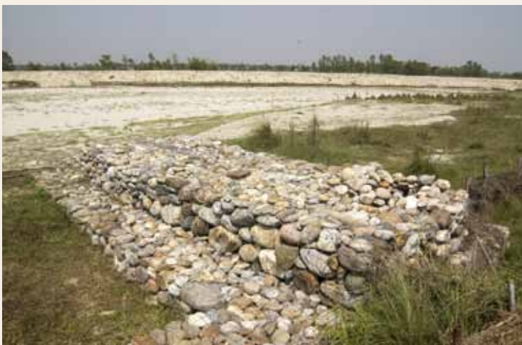
Spurs (use of stones and gibbon wire and plantation) seen near a river in eastern Nepal as a measure against floods. ©LWF Nepal
