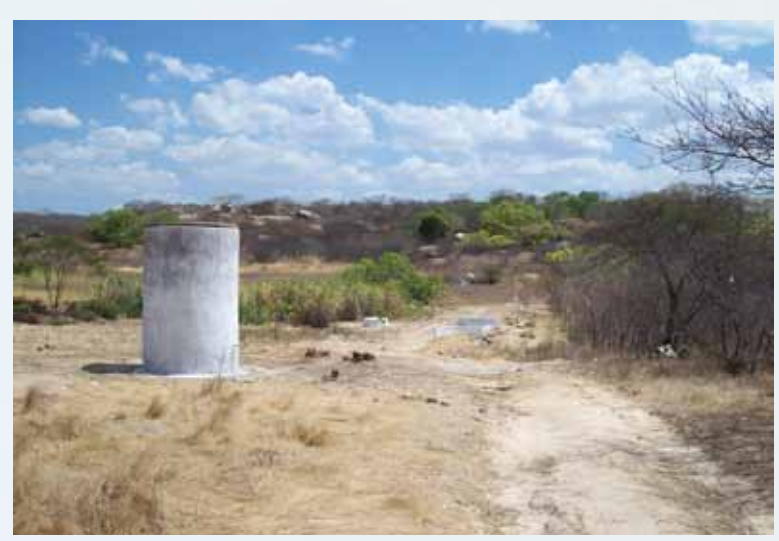
Water tank for irrigation purposes. Water is pumped into this above-ground circular cistern. With a controlled outlet at ground level, the force of gravity gives pressure for the farmer to release the water for irrigation purposes, using a long hose.
