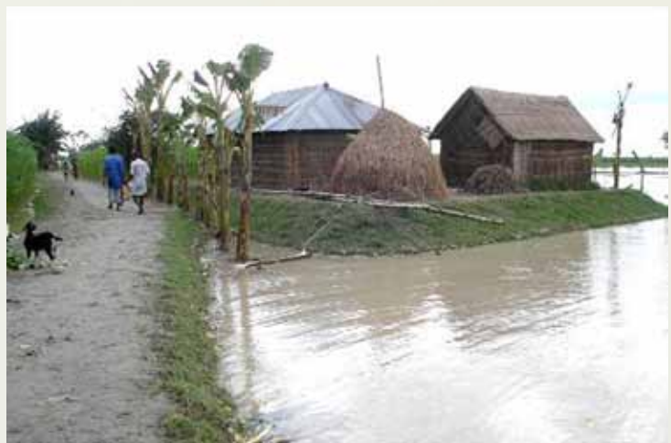
Homesteads raised some feet off the ground on improved plinth constructed by local communities (photos by Prodiapan)
