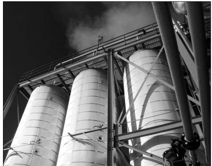
Ethanol Plant Photo: Aaron Brown
