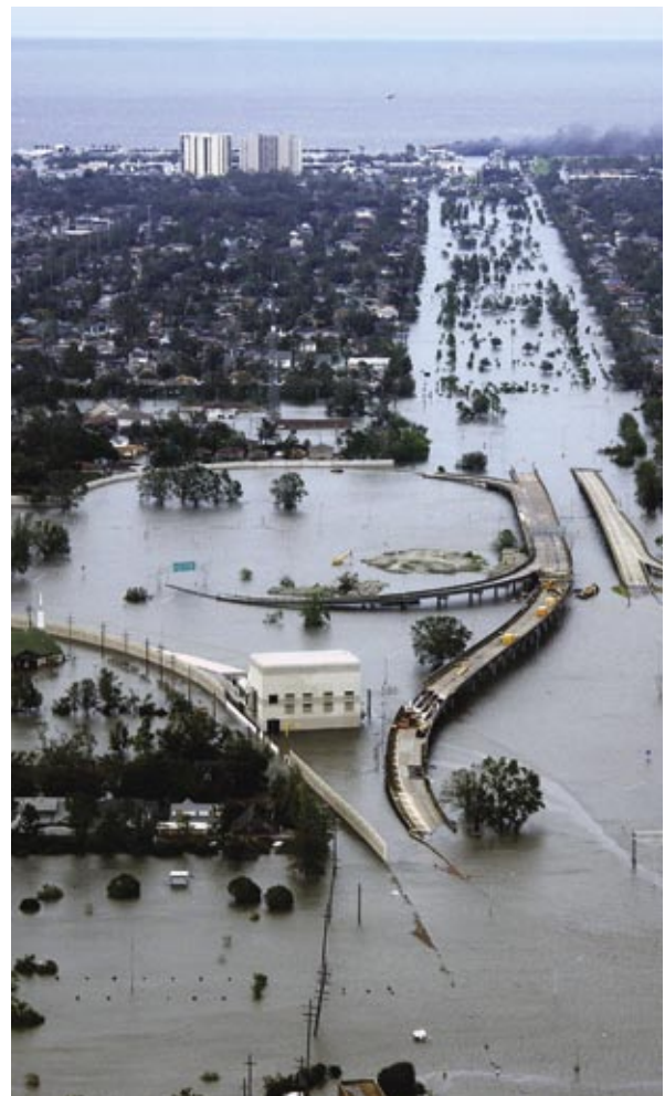
Flooding after Hurricane Katrina: one of 15 North Atlantic hurricanes in the record-breaking 2005 season.
