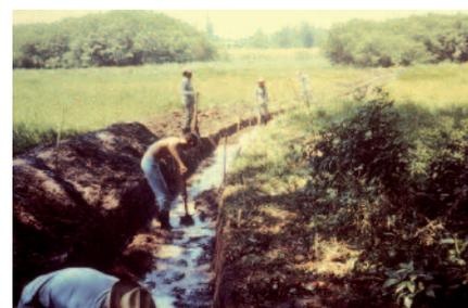
(Figure 5) Reconstructing a drainage canal in order to provide a permanent waterway promoting the free-flow of water through a malaria-prone (1981). Source: CDC
