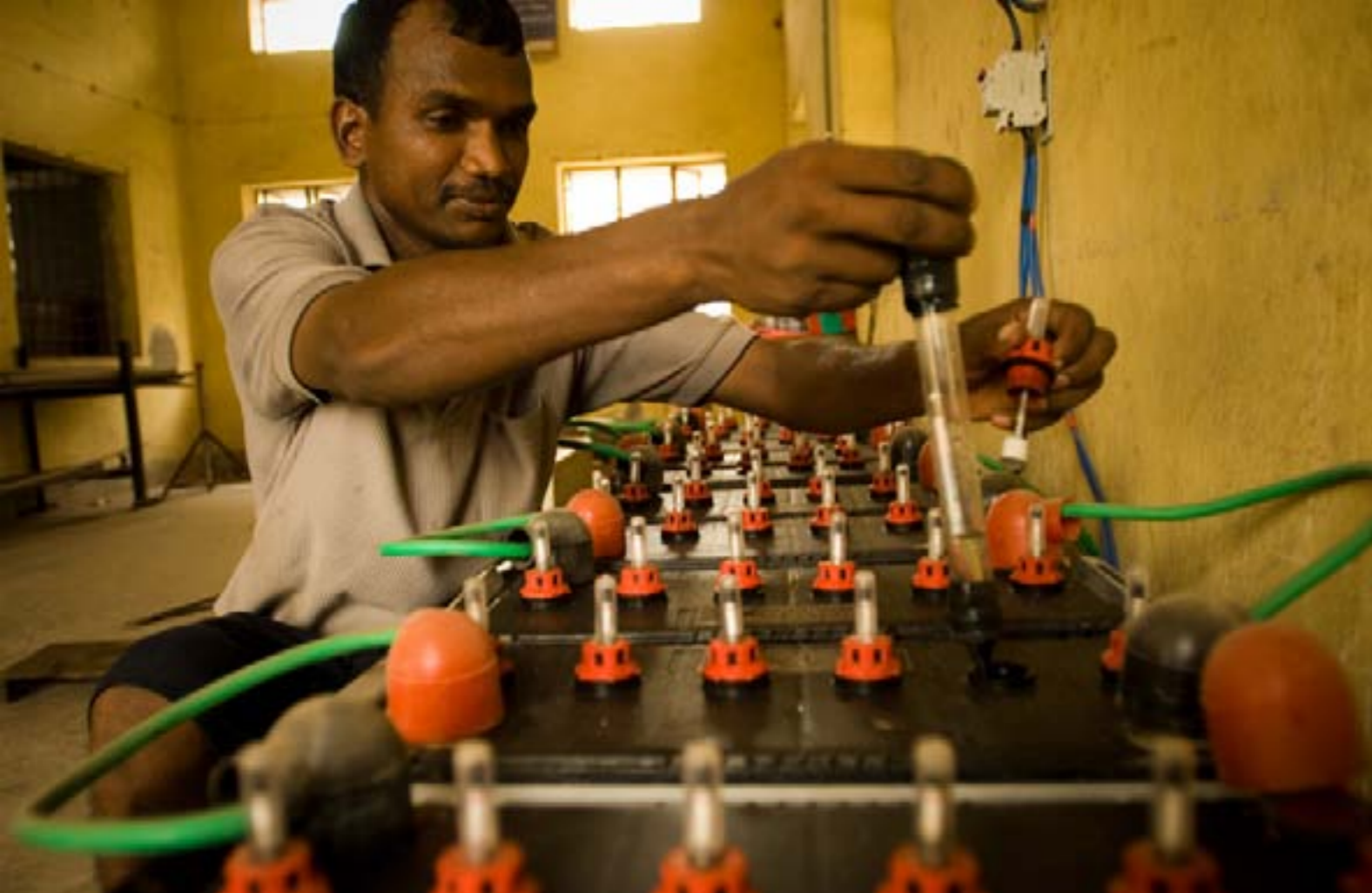
Image: Electrician Kosmos Bhakla measures the charging level of a battery bank in Solar Alternatives and Associated Programmes. The batteries are charged with electricity generated by solar photovoltaic panels on the roof. St. Mary's compound, Phulwaria Sharif, Patna, Bihar.
