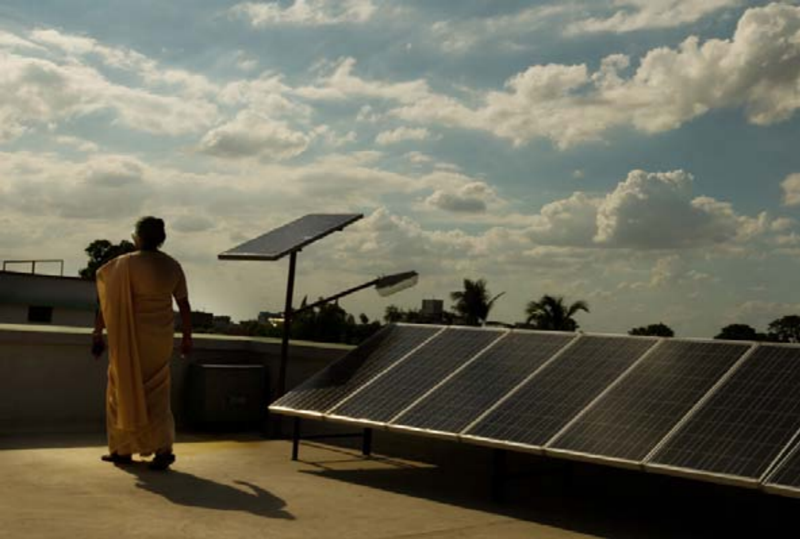
Image: Solar photovoltaic panels on the roof provide electricity to power lights, fans and computers in the building below. Tripolia Hospital, Patna.
