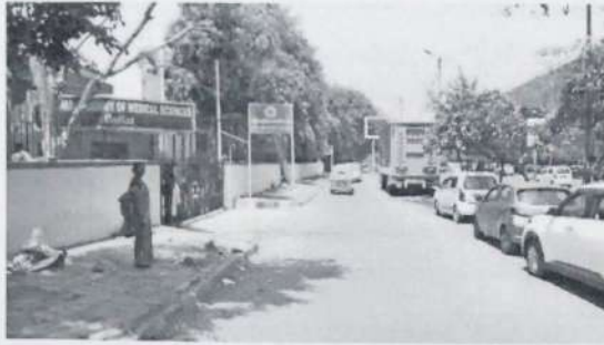
Image 3: Pavement condition of service road (Near Gate 6)
