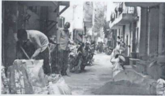
Image 15: Construction activities in Gautam Nagar Area
