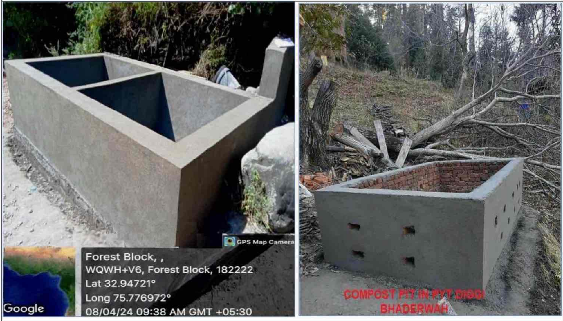
COMPOST PITS BEING CONSTRUCTED
