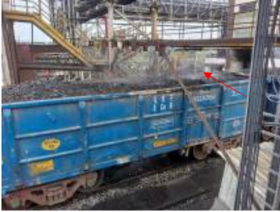
Water Sprinkling over Wagon (Pre-tipping)
