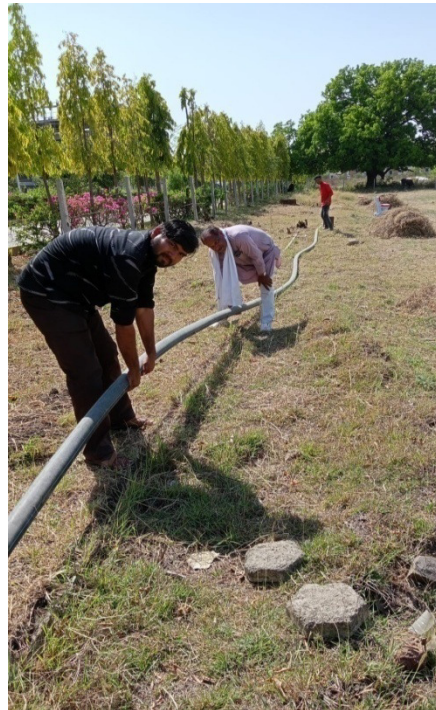
Dedicated pipeline laid for the reuse of treated wastewater in gardening purpose
