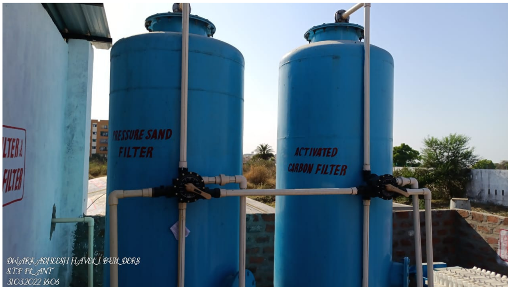
PSF & ACF installed at the back of STP Control room
