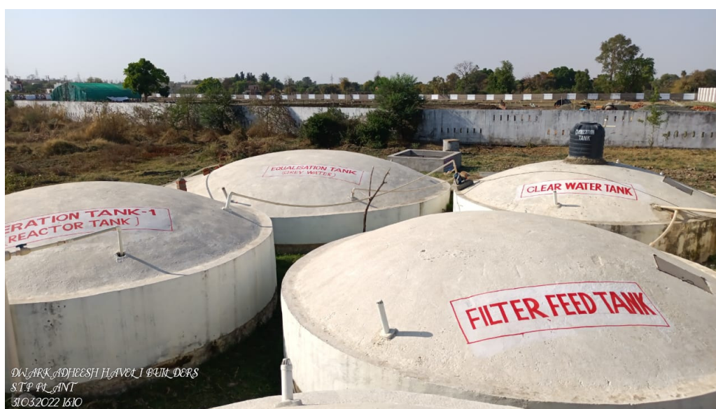
Various units of 250 KLD MBBR based STP
