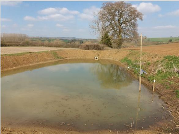
**Retention Ponds** are bespoke topographic depressions that provide additional storage capacity for floodwater and slow its flow into agricultural drainage systems and thus rivers. They are particularly common in the lower parts of agricultural fields
