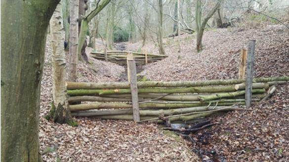
**Leaky Dams** are a flood mitigation technique in which logs are anchored across a stream to slow river flow. They store floodwaters upstream and encourage floodwaters to spill out of bank in low impact areas (such as forests and farmland) upstream of the assets at risk. There are many designs, most of which represent only a partial barrier.
