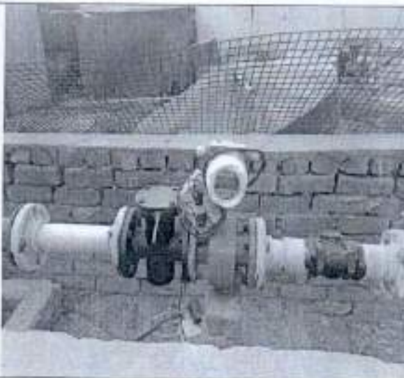
(c) Photograph of Tubewell No.3 with attached flow meter at Taj Hotel & Convention Centre, Agra.
