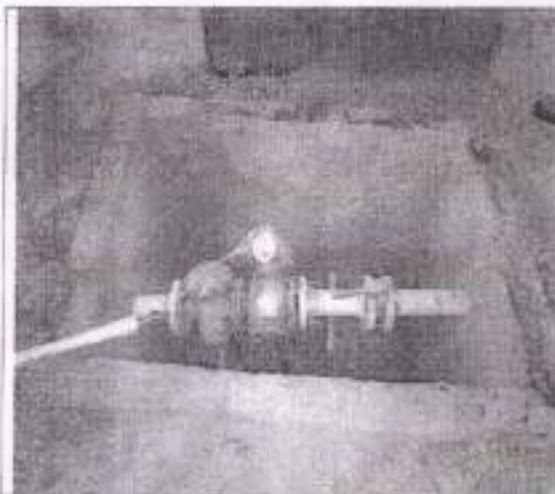
(a) Photograph of Tubewell No.1 with attached flow meter at The Oberoi Amar Vilas, Agra.
