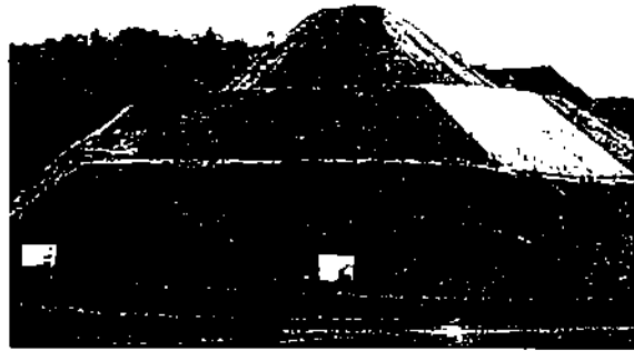
Required measures for dump management – retaining walls, drains and turfing
