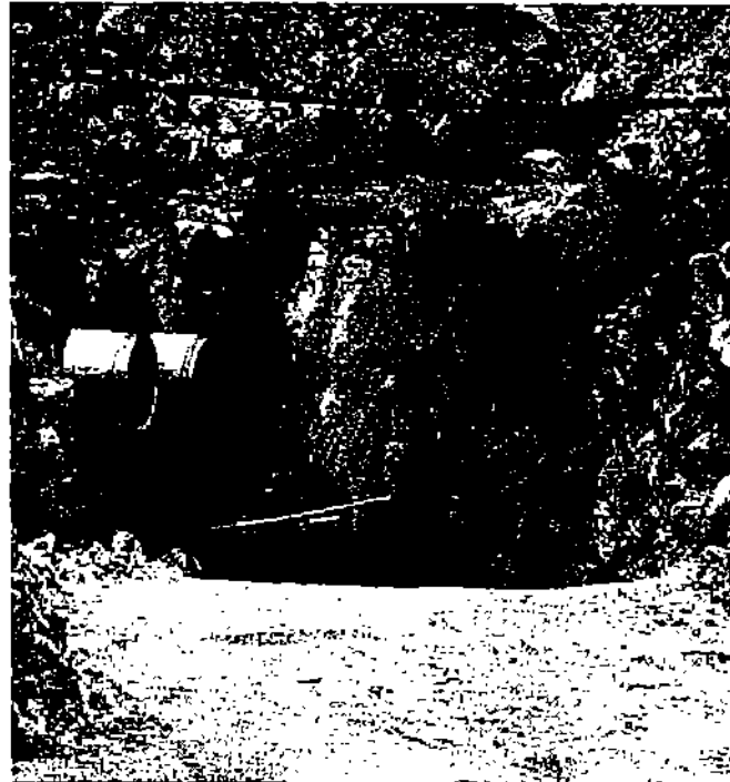
Provision made for circulation of oxygen to the tunnel
