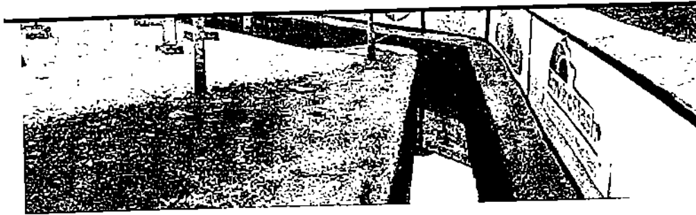
Photo showing dump management with retaining wall followed by garland drains at the to pumps.
