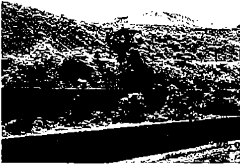
Required measures for dump management – retaining walls, drains and turfing
