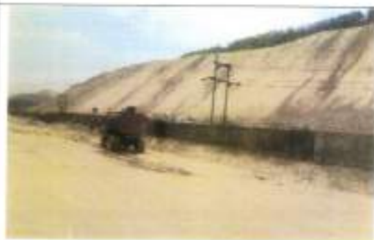
Retaining wall at the toe of dump
