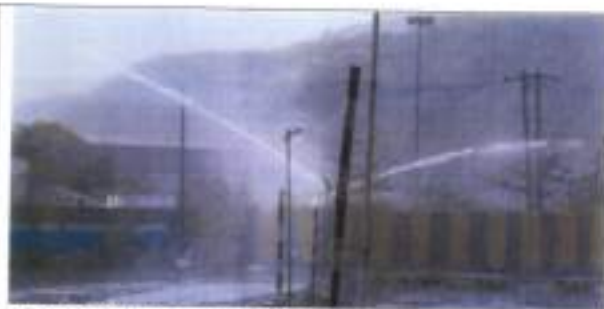
Fixed Sprinklers at coal Yard
