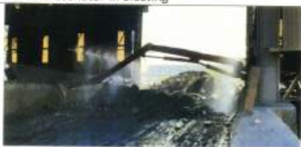
Water Sprinkling at Unloading Point at CHP (04 MTY)
