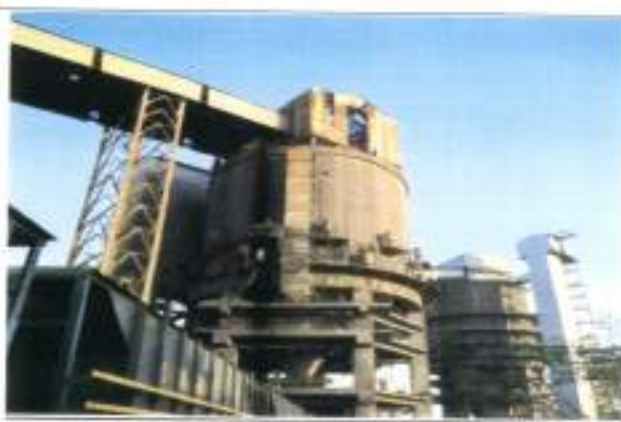
Loading of coal into wagons through Silo
