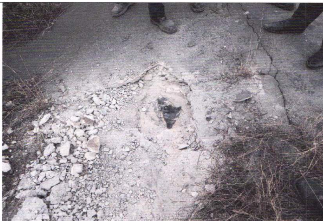
View of the HDPE liner provided on the bottom of the ash pond as per consent condition issued by MPPCB
