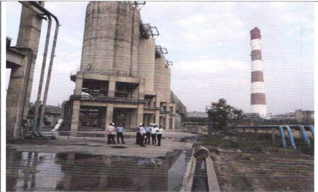
5 nos. of 1000 MT capacity each dry fly ash silos
