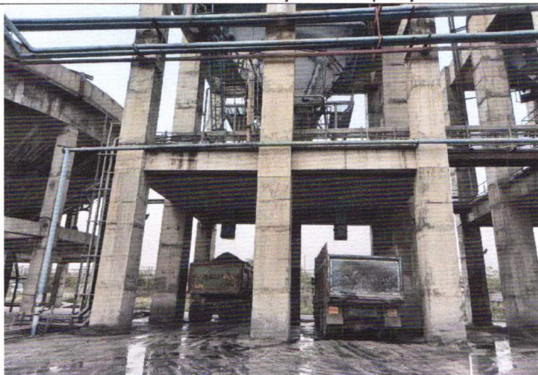
View of wet ash loading in trucks for disposing in low lying area
