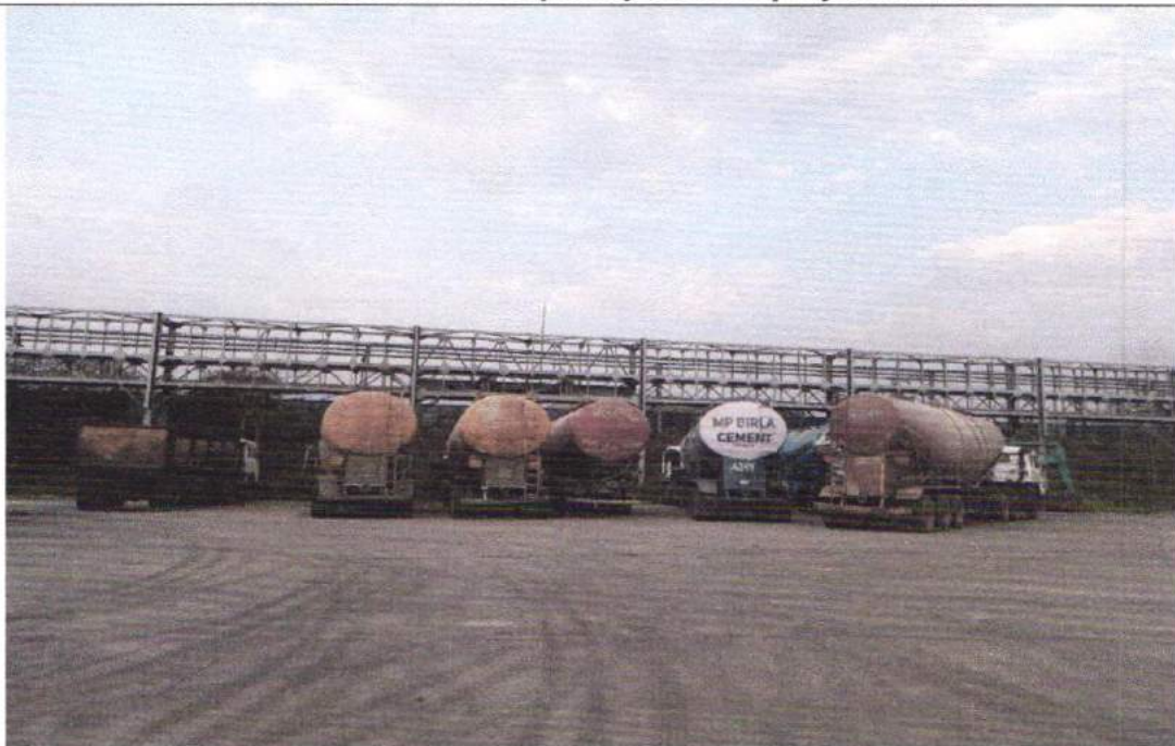
Dry ash transported to cement plants through bulkers
