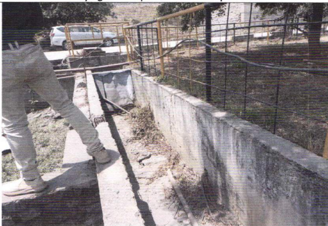
No wastewater discharged outside the plant. During visit the Plant and ash pond out let found dry
