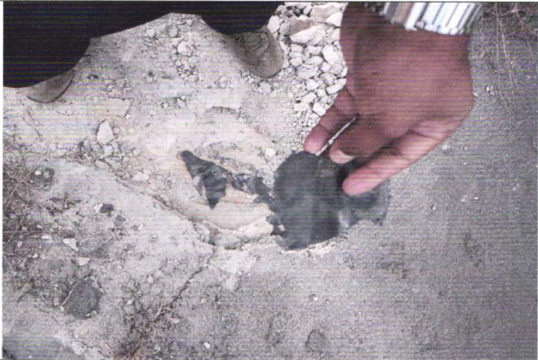
View of HDPE liner at the dyke of ash pond
