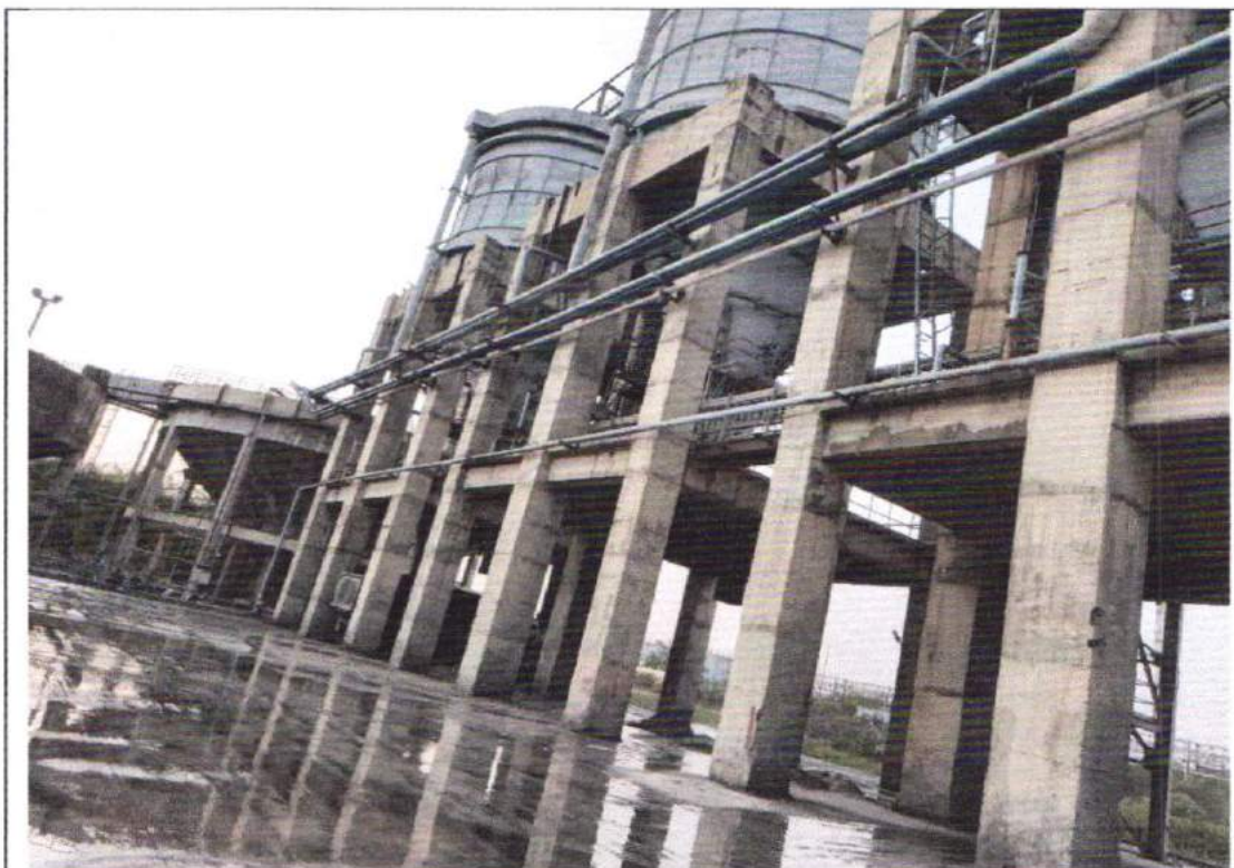
Bottom ash collected in 3 nos. of hydro bins capacity 750 MT each
