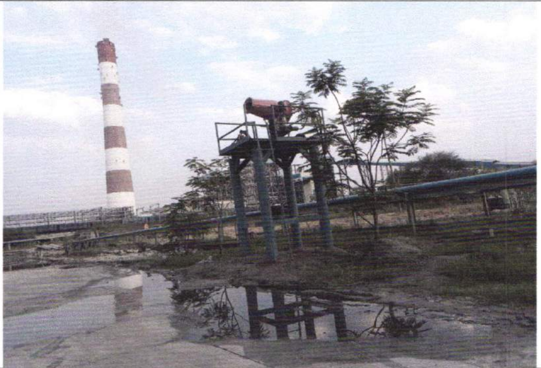
4 nos. of mist guns provided at the ash handling area to control fugitive emission due to vehicular movement on roads
