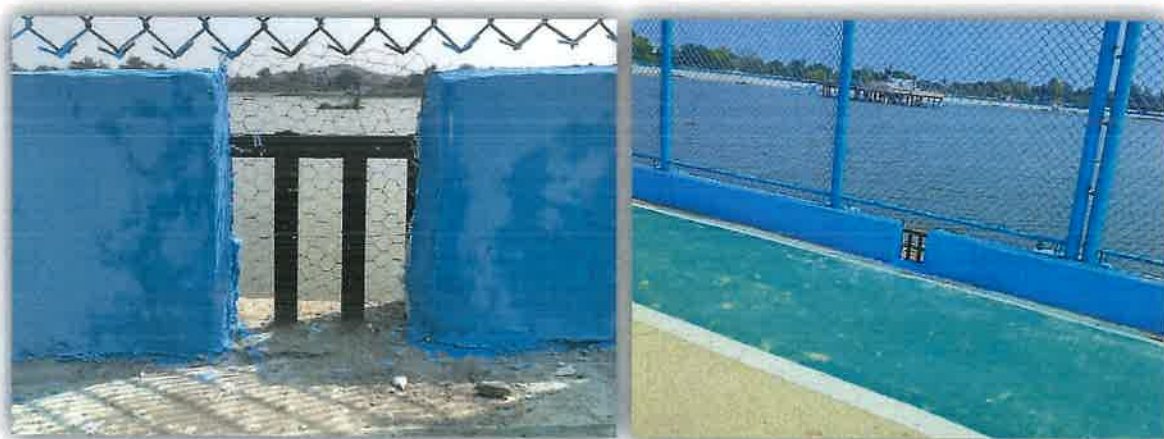
Figure 6: Fencing and 300mm x 230 mm hole in the wall
