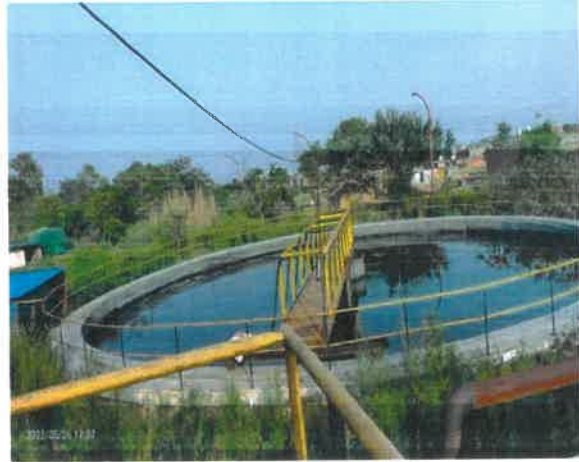
Fig.4: Secondary clarifier
