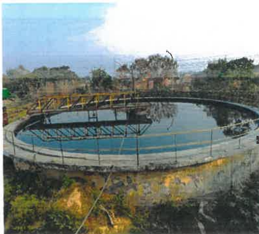
Fig.3: Secondary clarifier
