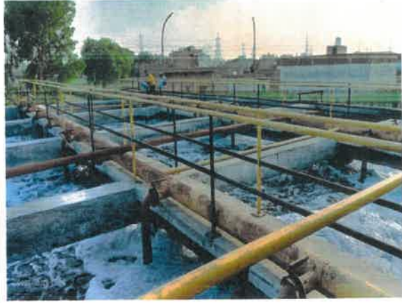
Fig.4: Aeration Tank
