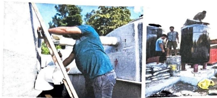
Placement, Fitting and Connection of Johkasou Tank and other equipments
