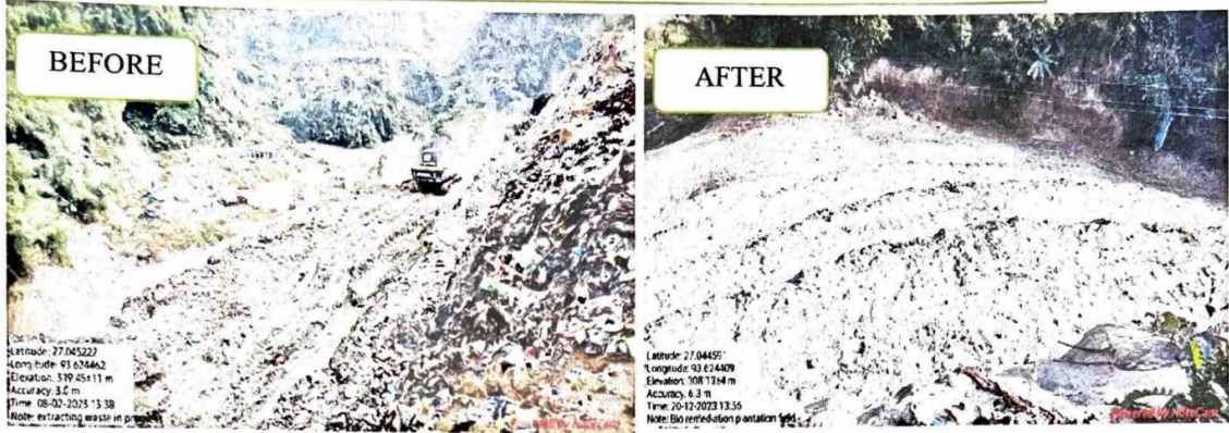
Extraction of Legacy waste at Chimpu site
