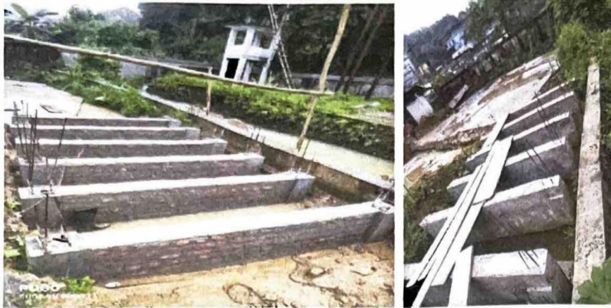
Construction of Foundation for STP Tanks
