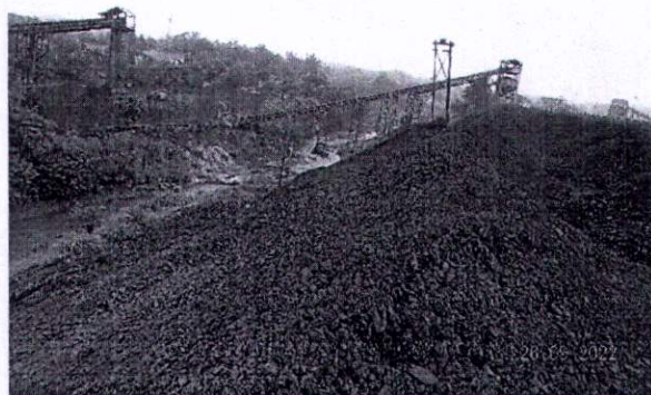
No catch drain , siltation ponds can be seen in between coal at the railway siding and river/nallah.
