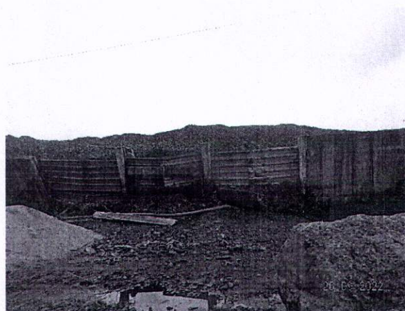
Photos 09& 10: Photos of temporary arrangement (metal sheet used) in place of broken wall in the north east direction of project. Coal dumps can be seen inside.
