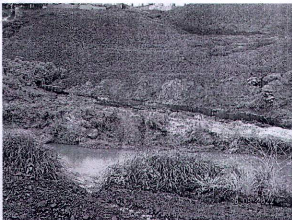
Photo 25: Photo of wall broken/coal breach and water coming from project wall sideto Sonadubi river.
