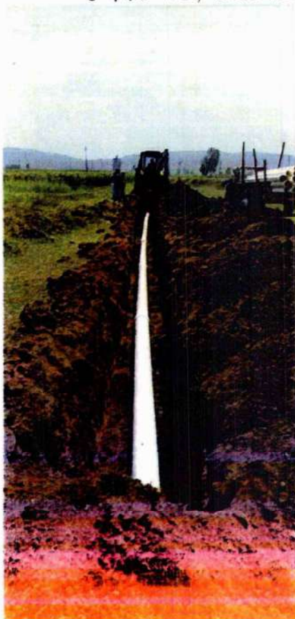
O PVC PIPELINE FITTING WORK IN PROGRESS
