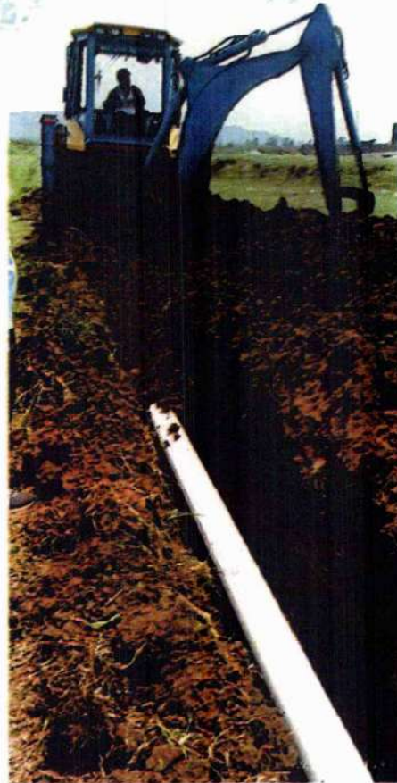
O PVC PIPELINE FITTING WORK IN PROGRESS
