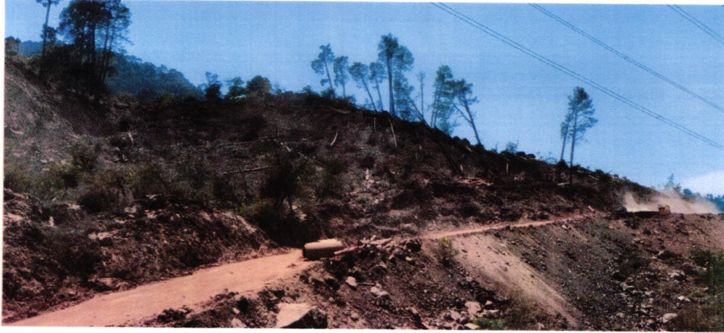
Fig.6. Field photograph illustrating slope and road affected by the landslide, with tilted and uprooted trees.
