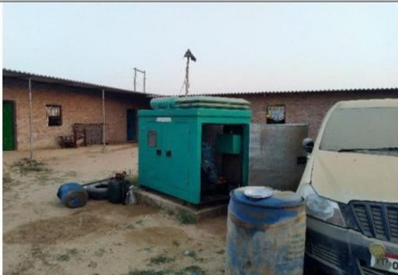
Fig. 13. DG Sets for Electric supply
