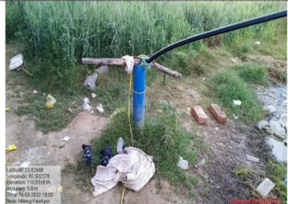
Fig. 12. Bore well for fresh water
