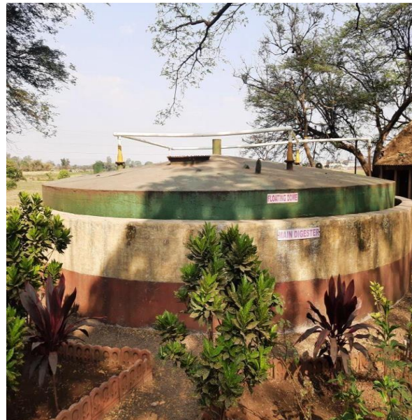
Photograph-4: A view of the 250 m 3 biogas plant for handling solid waste & liquid waste.
