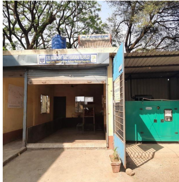
Photograph-6: DG set connected with biogas plant for source of electricity.
