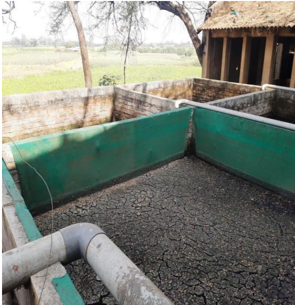
Photograph-5: Sludge drying beds.
