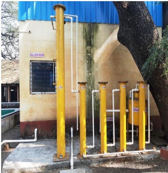
Photograph-7: Scrubbers installed for purification of biogas, prior to feeding for DG set.
