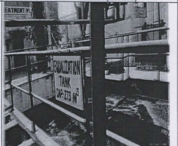
Pic-04. Equalization tank
