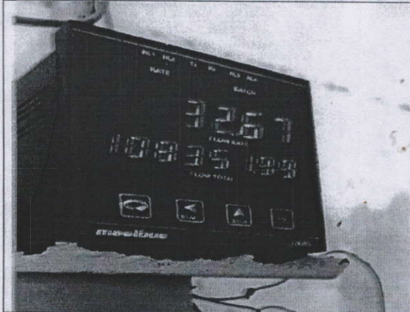
Pic-17. Display of discharge flow of treated effluent at ETP outlet
