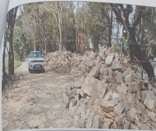
Building stone has been stored in the lake bed by BBMP(Lakes) contractor to construct diversion channel in order to prevent the entry of sewage/storm water into the lake
