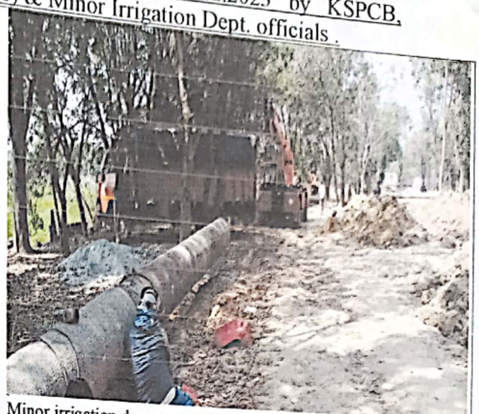
Minor irrigation department authorities are laying the steel pipe for conveying the treated sewage from Vengaiahnakere BWSSB STP to Yelemallappachetty lake pump house(Jock Well)
