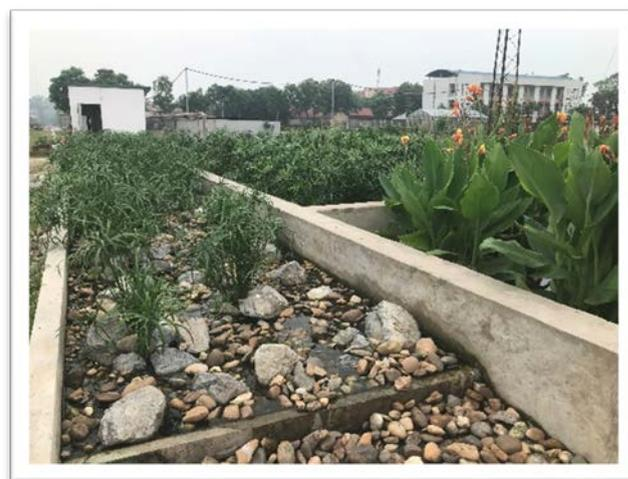
**Figure 2.** A decentralised wastewater system constructed in Hanoi, using nature-based technologies
