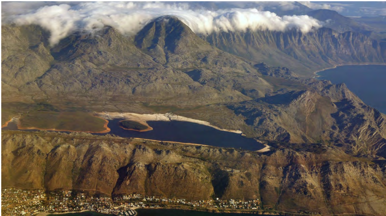
PHOTO 8C.1 Cape Town's Reservoirs
