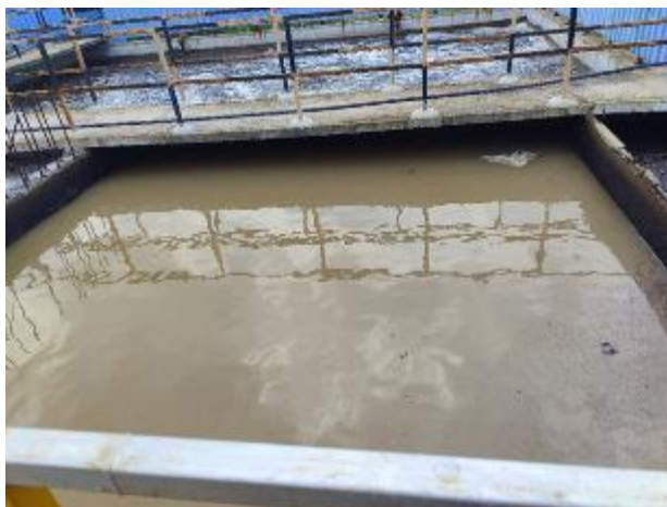
Secondary Clarifier and Neutralization Tank
