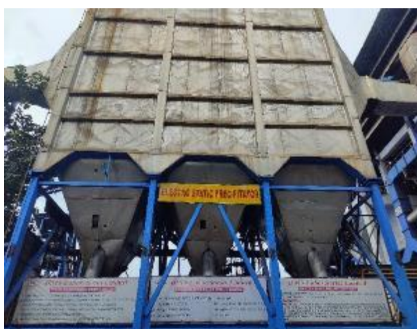
ESP followed by Stack Connected to Coal Fired Boiler
