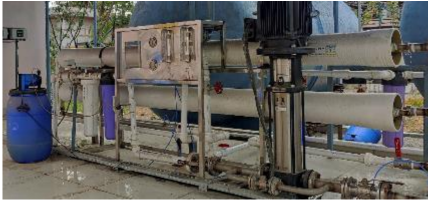
RO plant of 300 KLD Capacity
