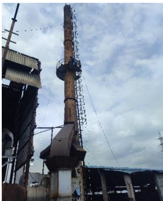
Stack connected to husk fired boiler
