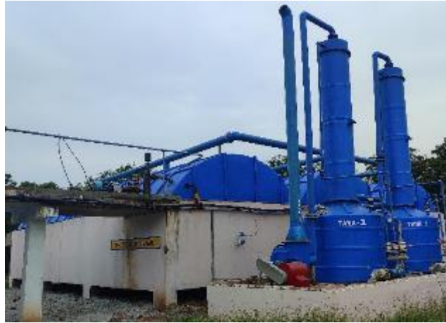
High TDS Effluent collection tank with Stripper
