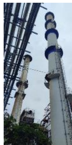
ESP followed by Stack Connected to Coal Fired Boiler
