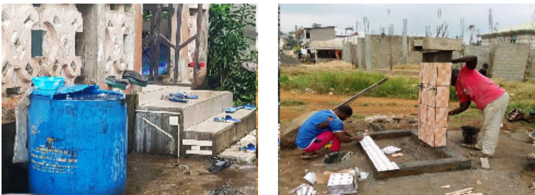
Figure 11. Rain Water Harvesting and construction of new stand taps as adaptation measure © Bryan Ngala
