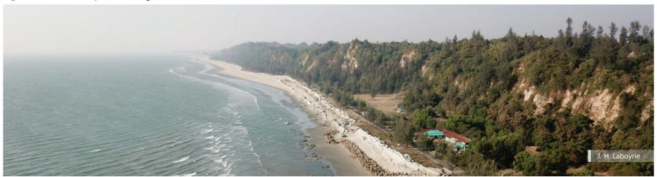
Birdseye view of coastal protection in Himchori: geotubes, randomly placed tetrapods, and a second series of geotubes along Marine Drive. *Source*: World Bank 2021a.
