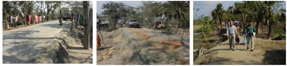
Damage to the landside slope of a coastal embankment from overtopping caused by Cyclone Sidr. *Photo credit:* Government of Bangladesh 2008 (first 2 photos); Islam et al. 2011 (right photo).
