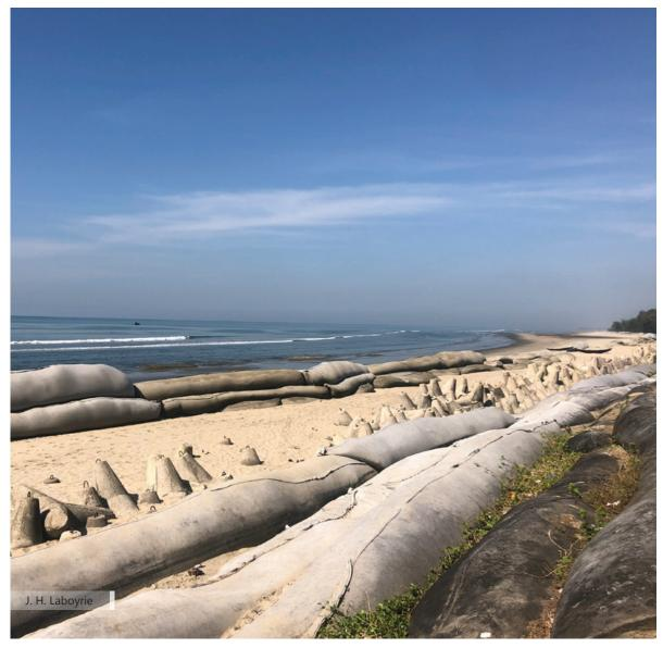
Seawall constructed with geotubes and tetrapods at Marine Drive.
