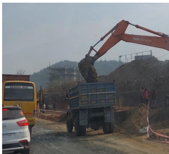
Figure 9: Uncovered Construction sites
