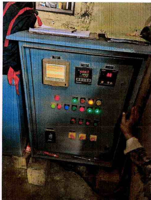
Control Panel for Methane Flaring
