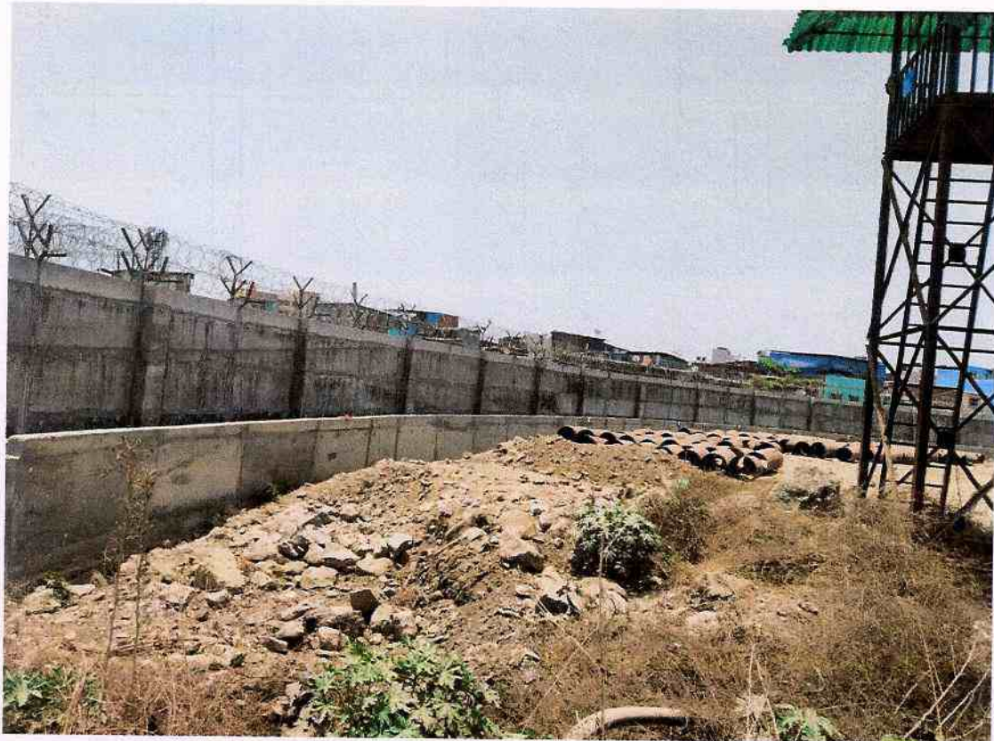
RCC Boundary Wall with Barbed Wire Fencing towards residential area at Deonar Dumpsite
