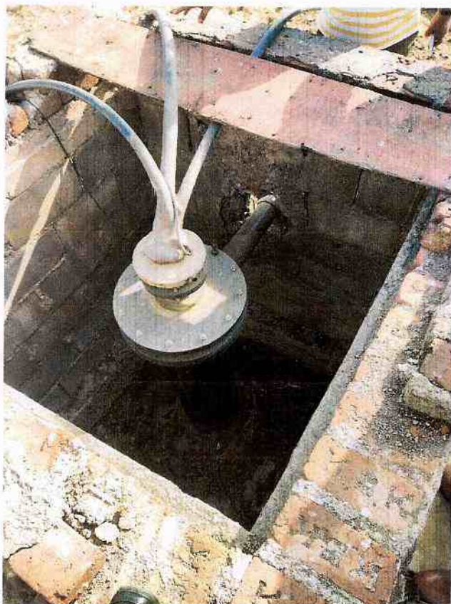
Gas Well for Methane and Leachate Collection
