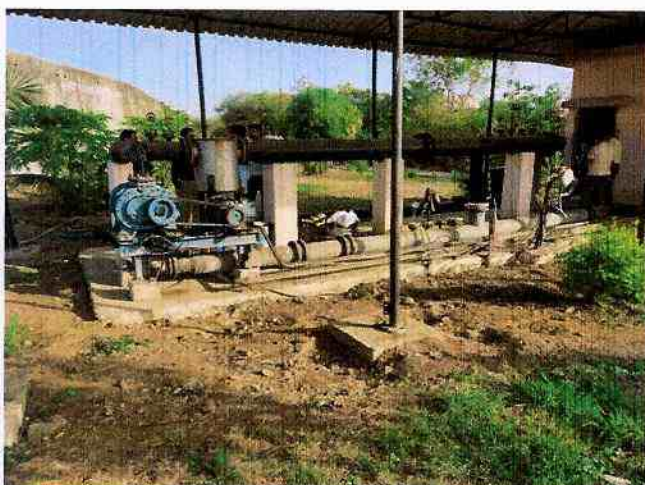
Methane Pumping System at Flaring Station
