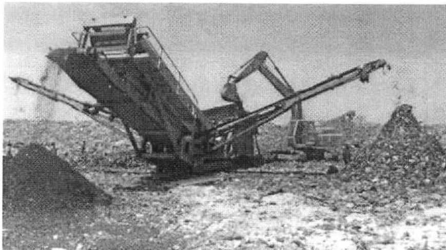
Img-4: Mobile Screen screening the existing Dump at Site
