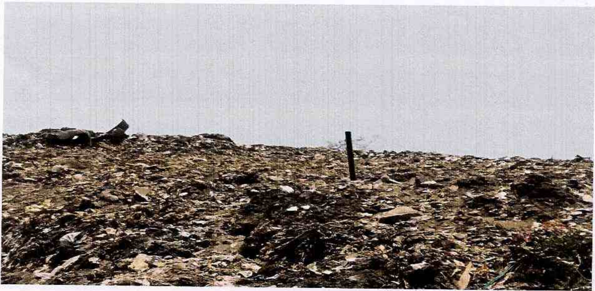
Perforated HDPE Pipes of 6 meter length inserted at Deonar Dumpsite
