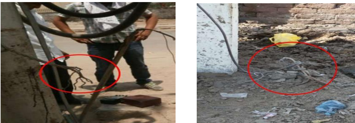
Figure 9: Improper Earthing Connection
