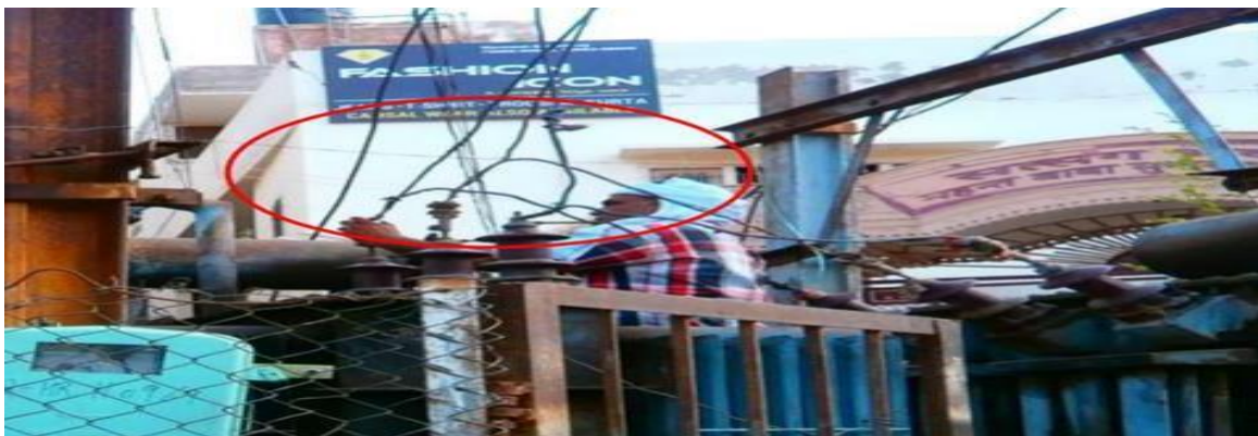
Figure 3: Single go switch for multiple DTs
