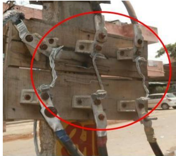
Figure 13: Installation of inappropriate rating & size of fuses
