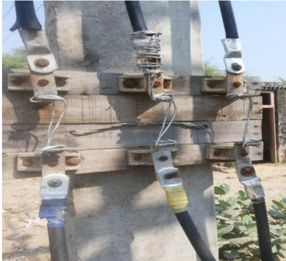
Figure 13: Installation of inappropriate rating & size of fuses
