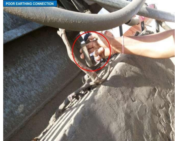
Figure 10: Improper rating of earth wire
