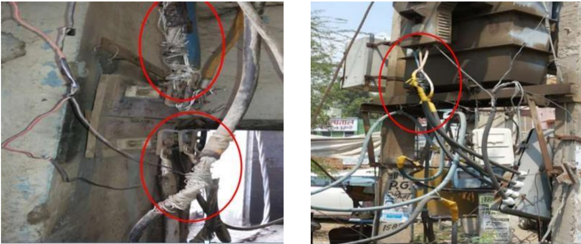
Figure 8: Loose jointed LT Leads
