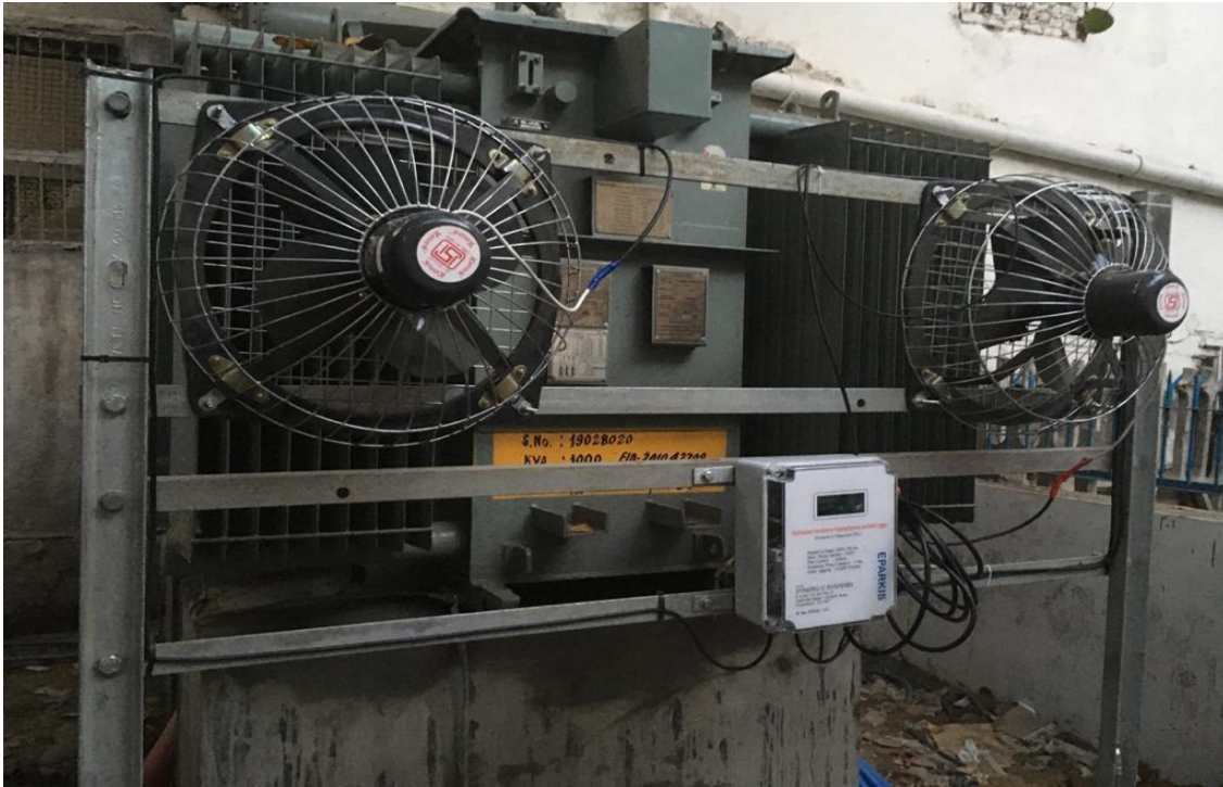
Plinth mounted DT with auto cooling system
