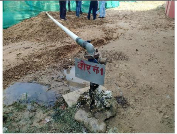
Fig. 14. Bore well at Washing Unit
