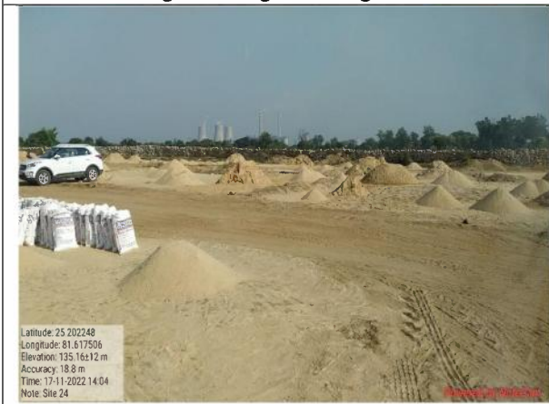
Fig. 27. Storage of Finished Materials
