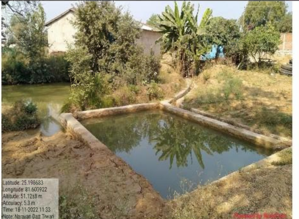
Fig. 4. Effluent Treatment Plant at Washing Unit
