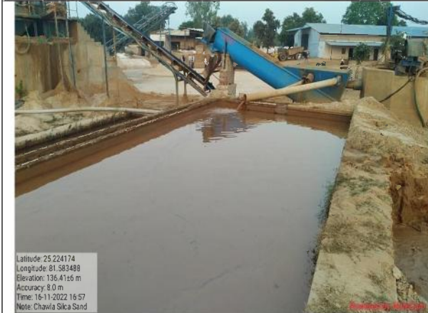
Fig. 3. Effluent Treatment Plant at Washing Unit
