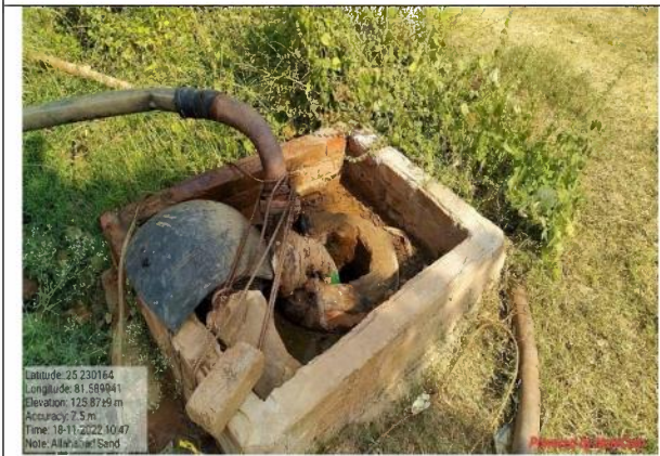
Fig. 11. Bore well at Washing Unit
