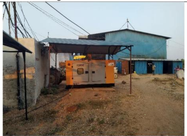
Fig. 18. Installed DG set
