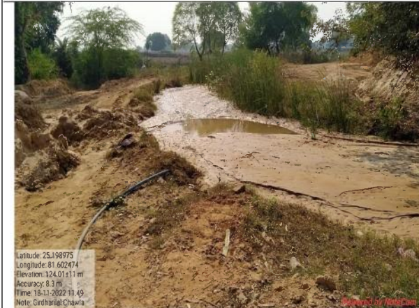
Fig. 5. ETP Sludge Disposal
