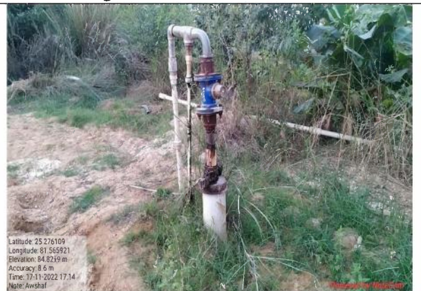
Fig. 12. Bore well at Washing Unit
