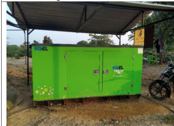
Fig. 17. Installed DG set
