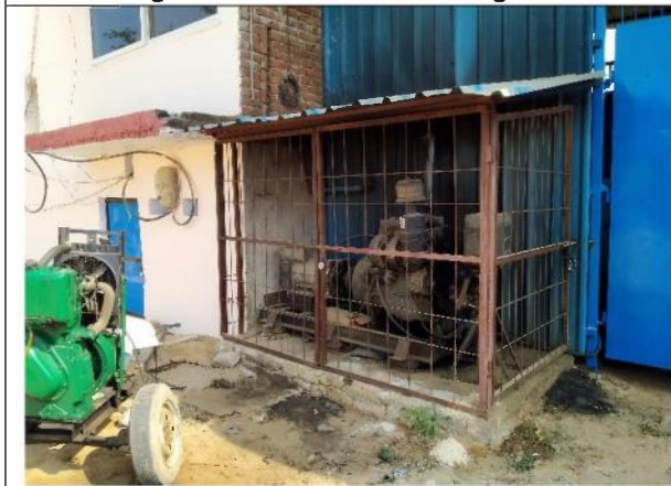
Fig. 15. Installed DG set
