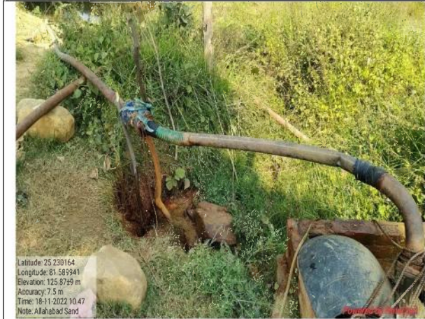
Fig. 13. Bore well at Washing Unit
