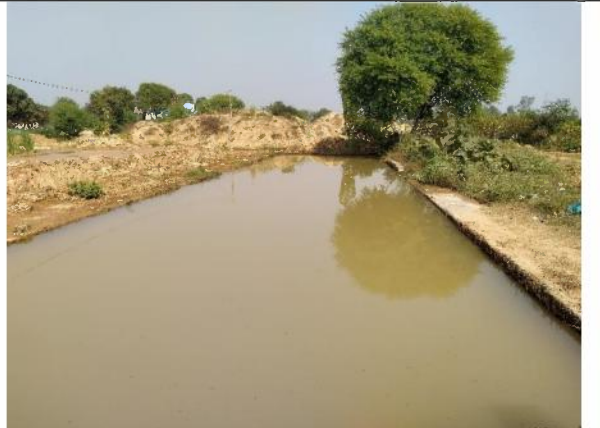
Fig. 2. Effluent Treatment Plant at Washing Unit
