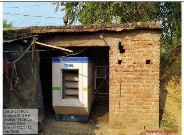
Fig. 16. Installed DG set
