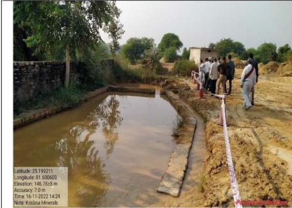
Fig. 1. Effluent Treatment Plant at Washing Unit
