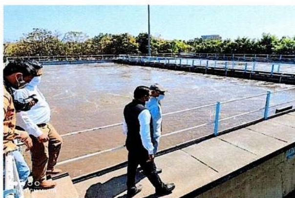
Plate: 8 : Aeration tank of Activated Sludge Process
