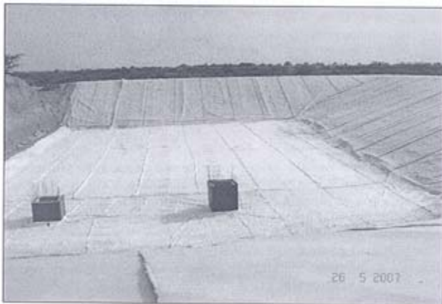
SLF under construction at TSDF Kumbhi, Kanpur Dehat
