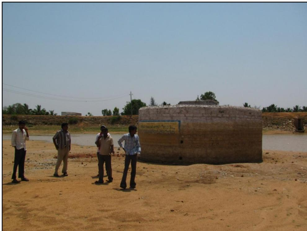
**Photo 8:** The structure of a recharge borewell located in a tank
