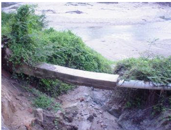
Photo 3. Damage caused by the Bañaderos river – Honduras.
