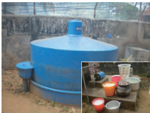
Fig. 8 A decentralised anaerobic digestion in Kerala, India
