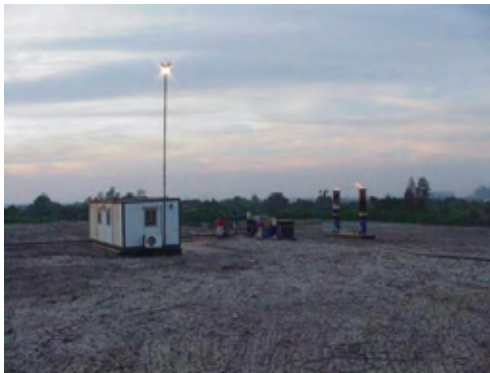
Fig. 11 Sanitary landfill with gas recovery system in Thailand (Photo: Komsilp Wangyao).
