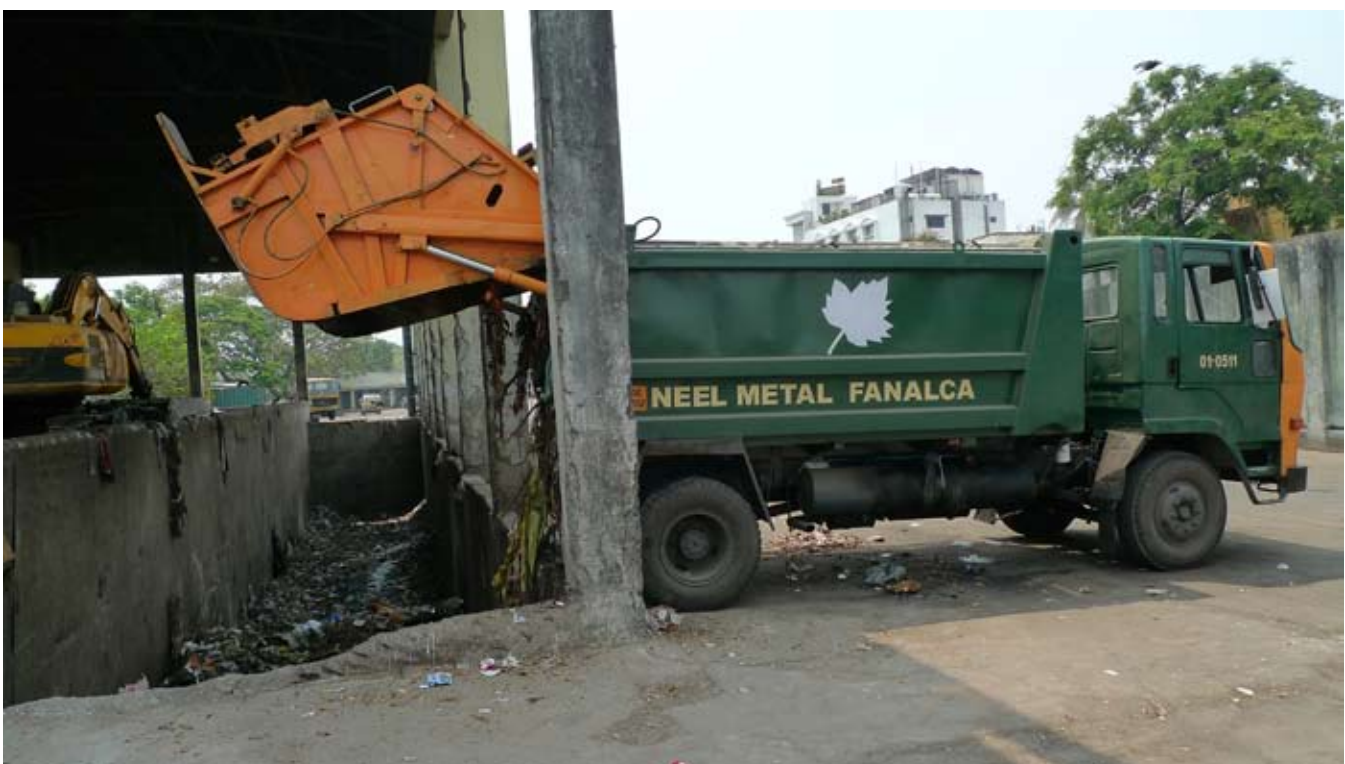
NEEL METAL FANALCA TRANSFER STATION, KODAMBAKKAM, CHENNAI
