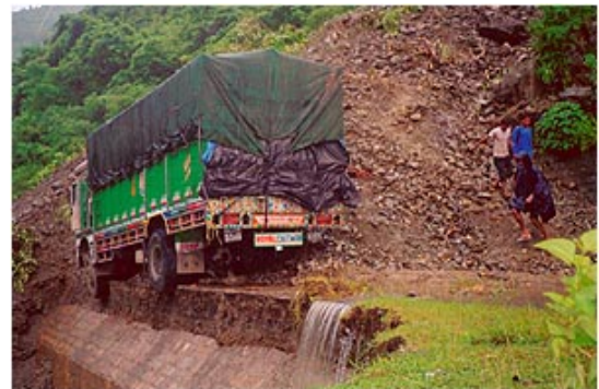
Figure 5 Landslide at Naubise road
