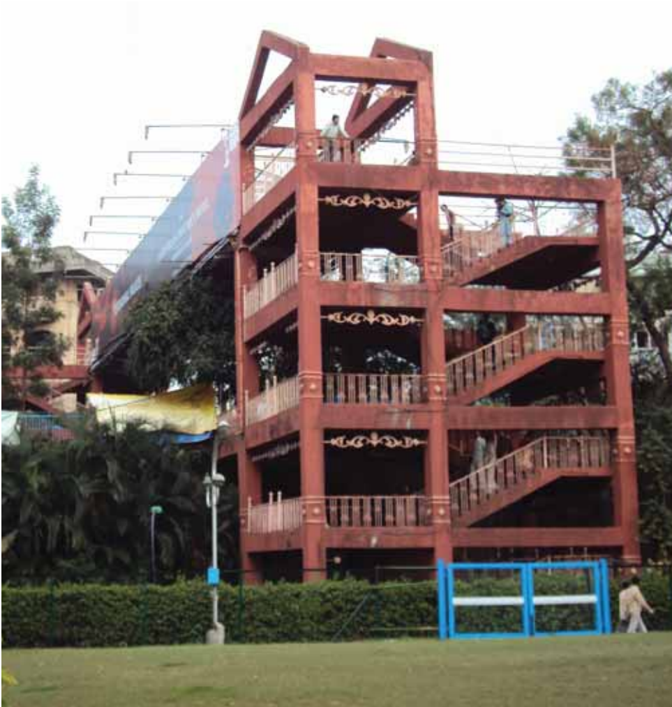
FOB at Sarasbaug - like climbing 4 floors!
