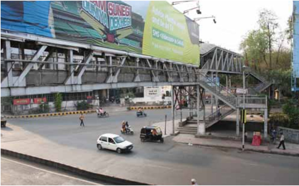
This photograph shows the massive size of the FOB on Karve Road, outside the SNDT College.
